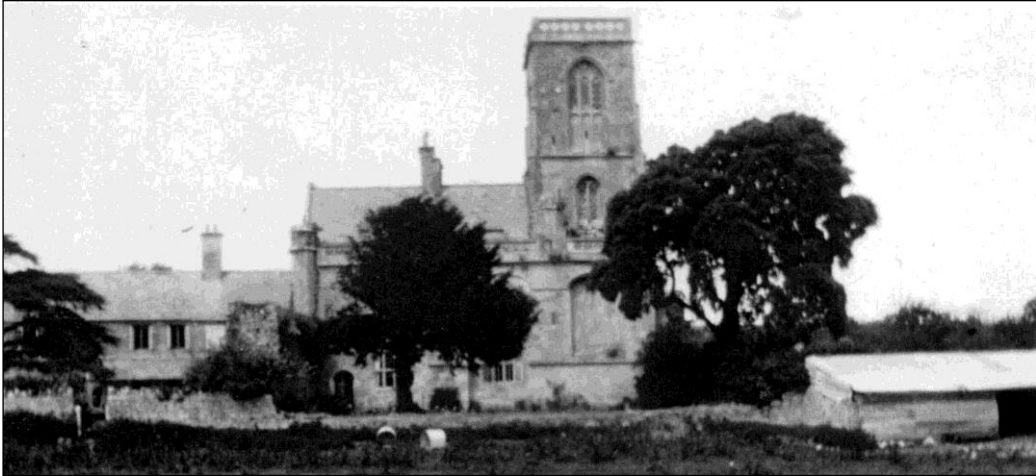
Figure 21. View of south front of the former church and farmhouse in ?c.1890.
