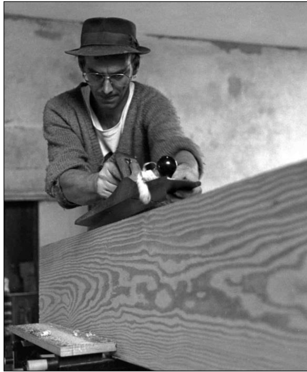
Figure 42. Planing a new floor board.
