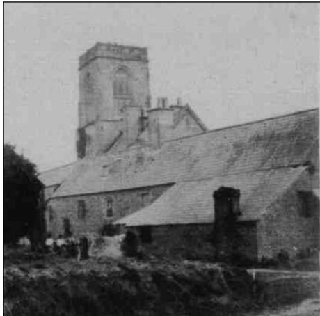
Figure 19. A lean to against the north elevation of the 1701 farmhouse.
