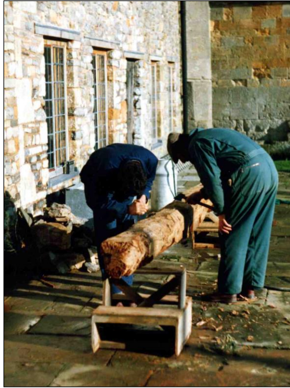
Figure 37. Repair of a ceiling beam.
