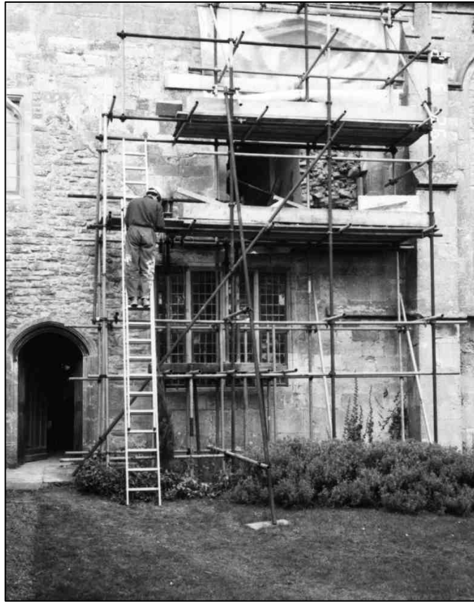
Figure 40. Scaffolding erected around the exterior of the window, (south elevation)
