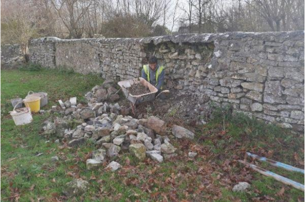
Rebuilding the walls at Woodspring in 2020.
