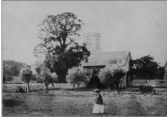
Figure 18. View of church tower with infirmary in foreground.
