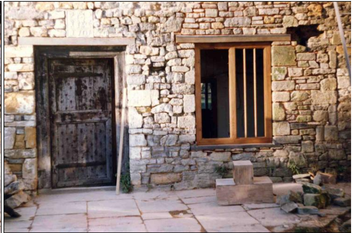
Figures 32 & 33. Farmhouse windows and door being replaced.
