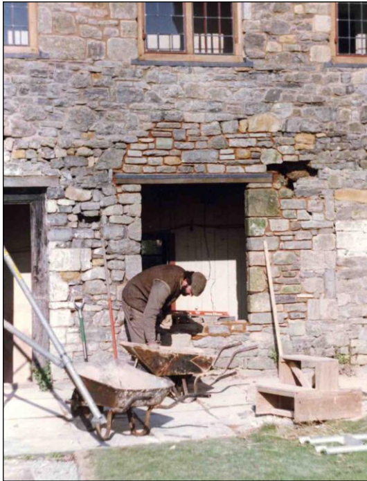
Figures 32 & 33. Farmhouse windows and door being replaced.
