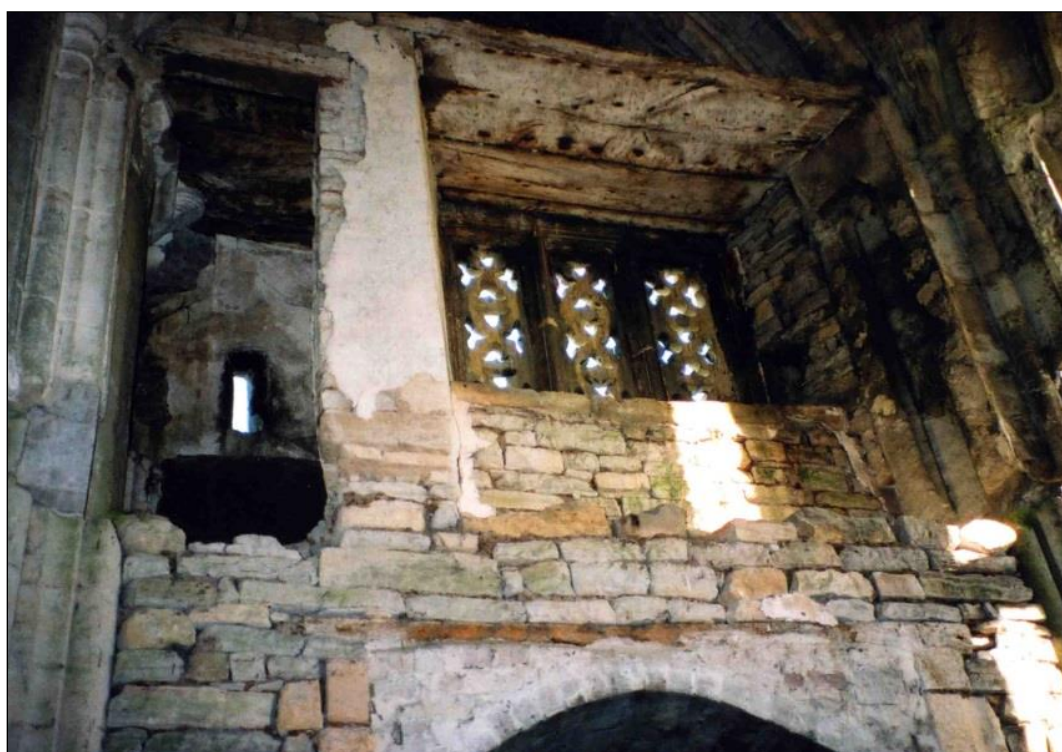
Figure 11. Upper part of east wall in crossing. Note the remains of the latrine on the left.
