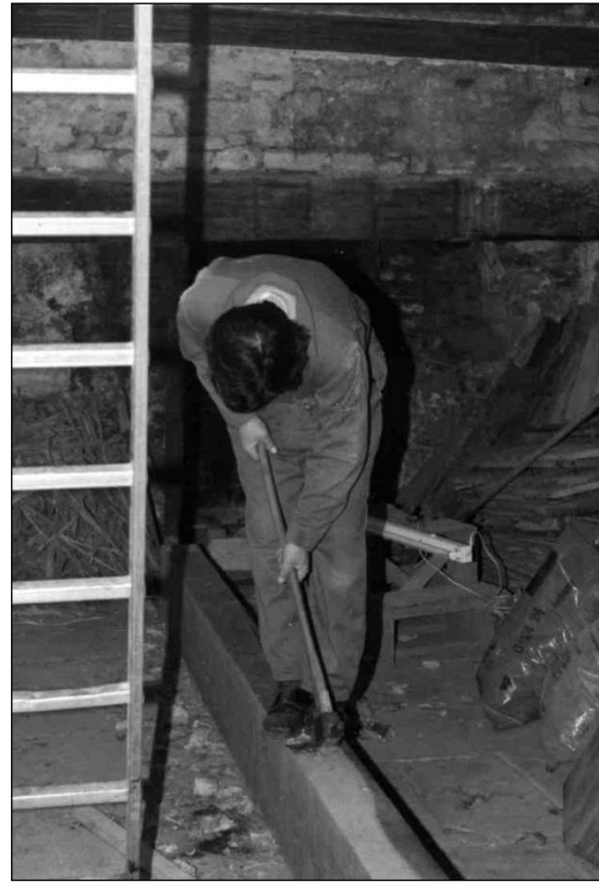
Figure 46. Mike Haycraft using an adze, a tool in use since the Middle Ages.
