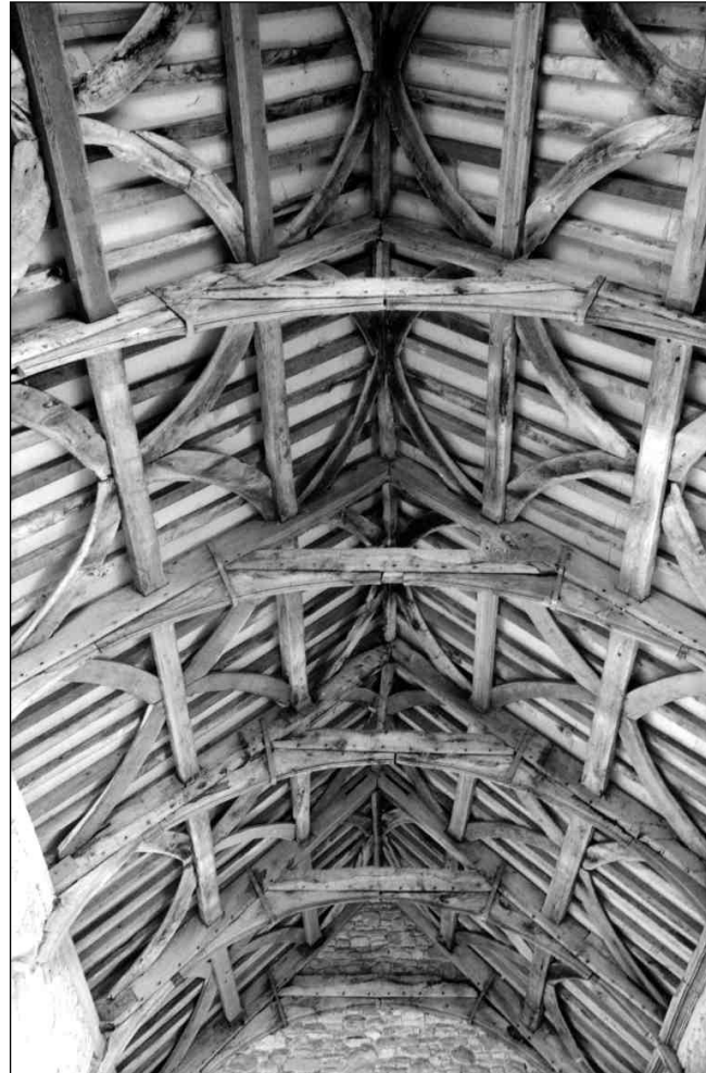
Figure 9. Interior of Infirmary, after the 1987 restoration of the roof.
