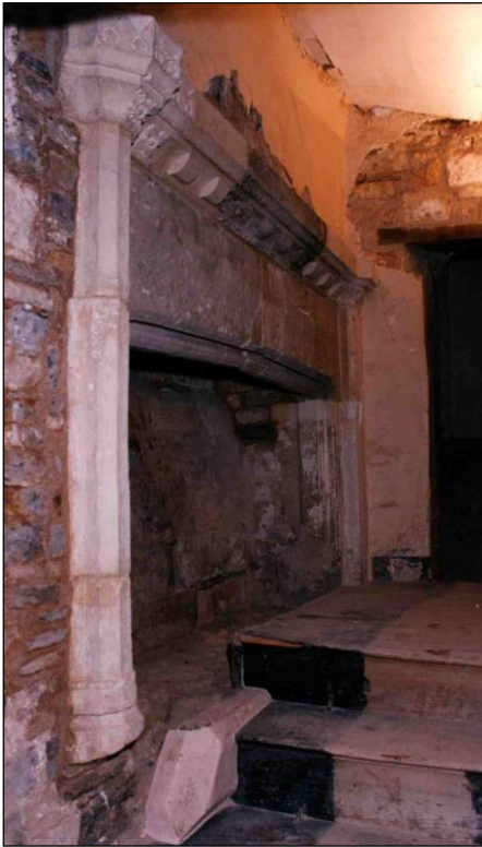
34 Figure 34. Reconstructed fireplace in first floor bedroom.
