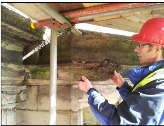
Examples of stonework decay and damage. Some of the 1970s cementitious repairs, like the plinth bottom right, had stood up well. In such cases, there was no need to replace.
