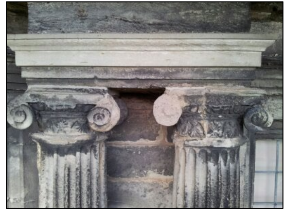
Examples of stonework decay and damage. Some of the 1970s cementitious repairs, like the plinth bottom right, had stood up well. In such cases, there was no need to replace.
