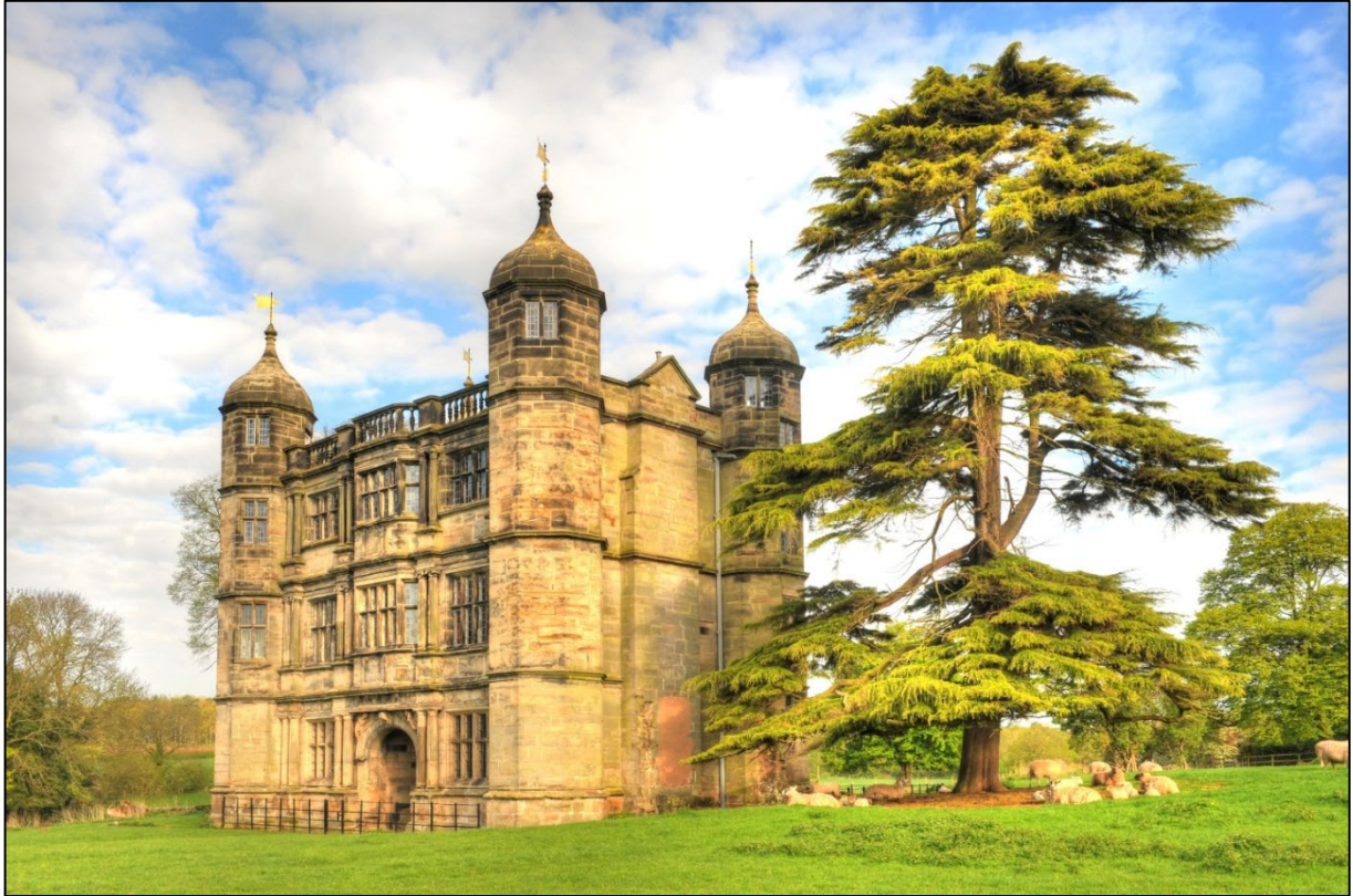
Tixall Gatehouse after the 2012 stone repairs, with all four weathervanes flying once again. Each vane bears a number, to make up the year '1976', when the first restoration was completed.
