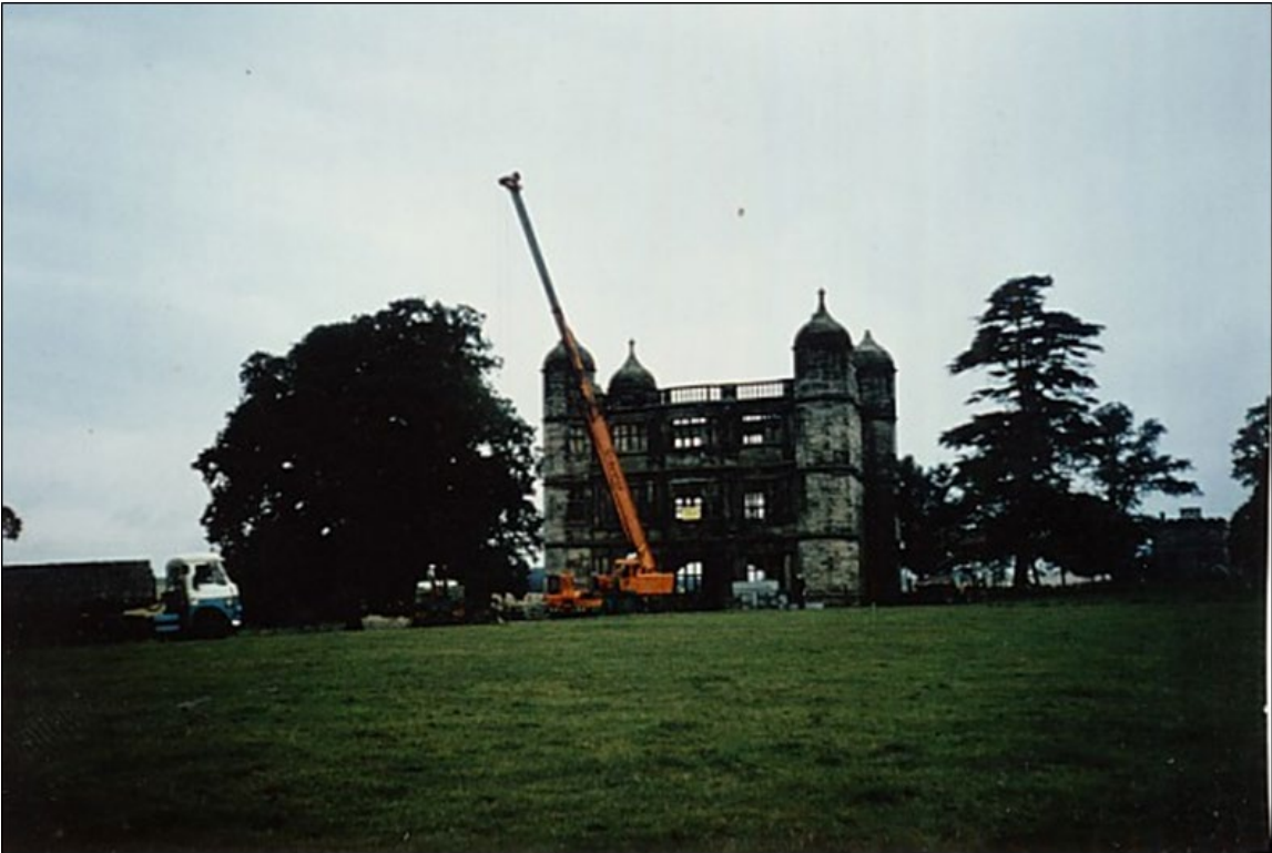
A crane was used to lower materials into the building, to avoid having to use the narrow staircases.
