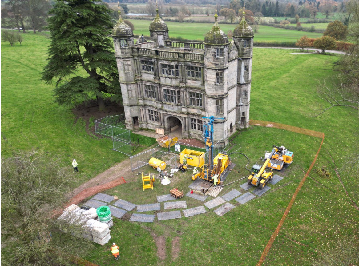
Drilling the boreholes for ground source heat capture in Jan 2025, and the hatch, thoughtfully installed in initial 1970s restoration and invaluable for hoisting building materials and furniture alike.
