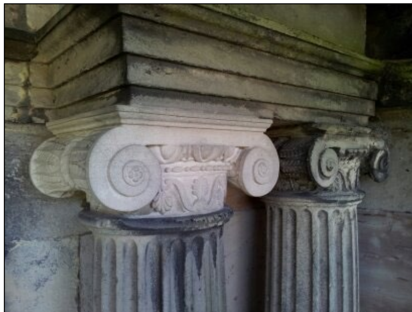
One of Mr Walker's 1970s capitals, standing up well to the passage of time.
