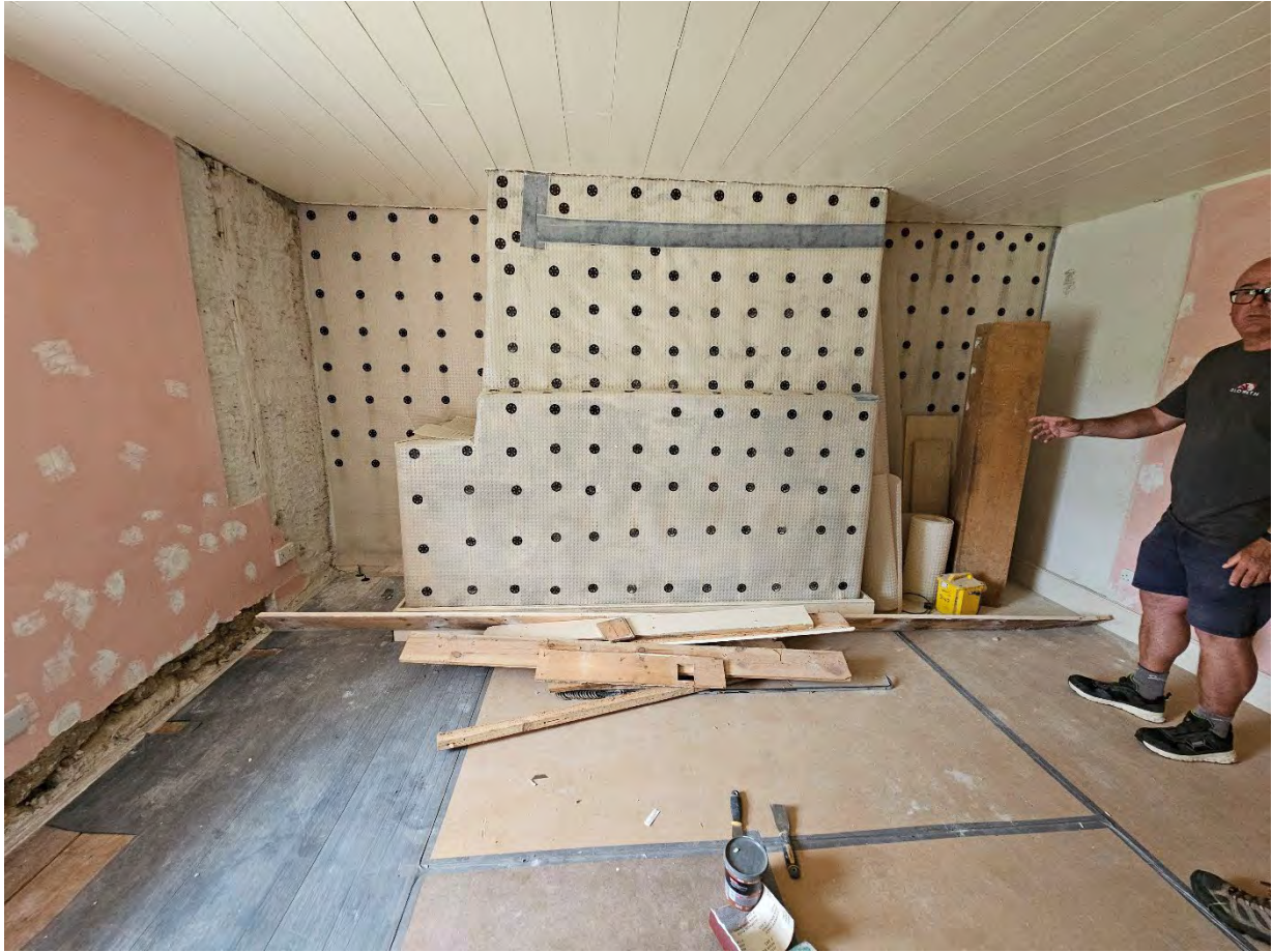
The Farmhouse first-floor west chimney breast under repair with insulation ready to receive lime plaster (below).
