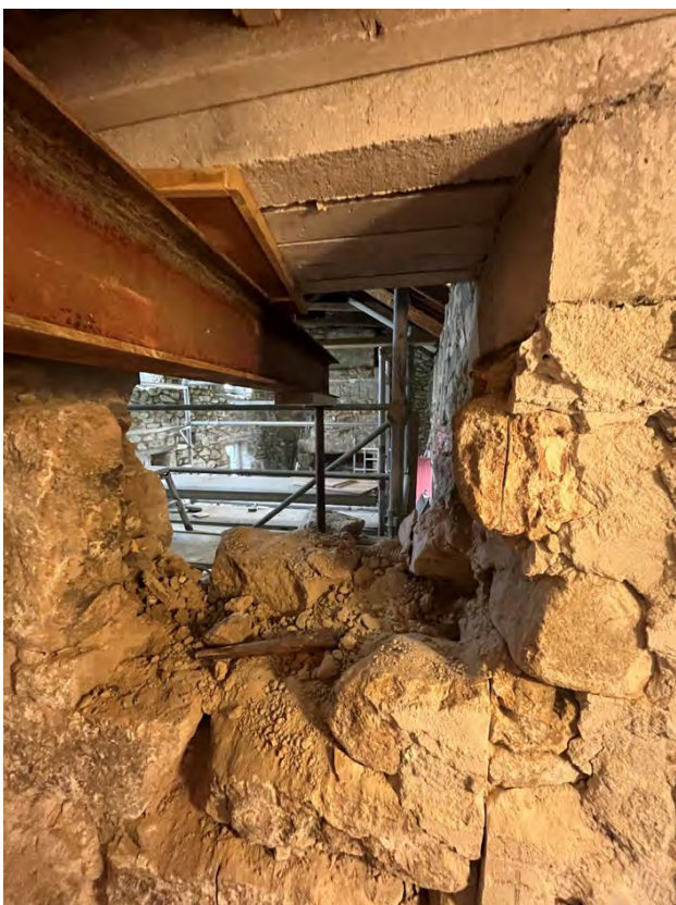
Breaking through from Captain's House to the barn cottage and the creation of the new interconnecting doorway.
