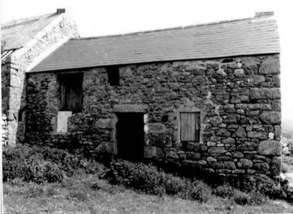
Captain's Barn in 1988, revealing its many adaptations for agricultural use. These openings were subsequently blocked. National Trust Vernacular Survey 1988.
