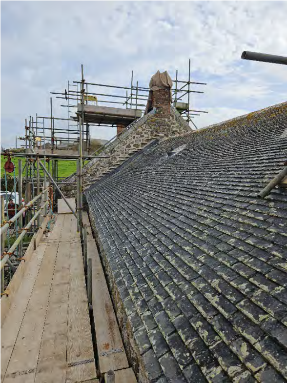
Repairs underway to the chimneys and scantle roof of Captain's House, and the repointed west wall of the barn end.
