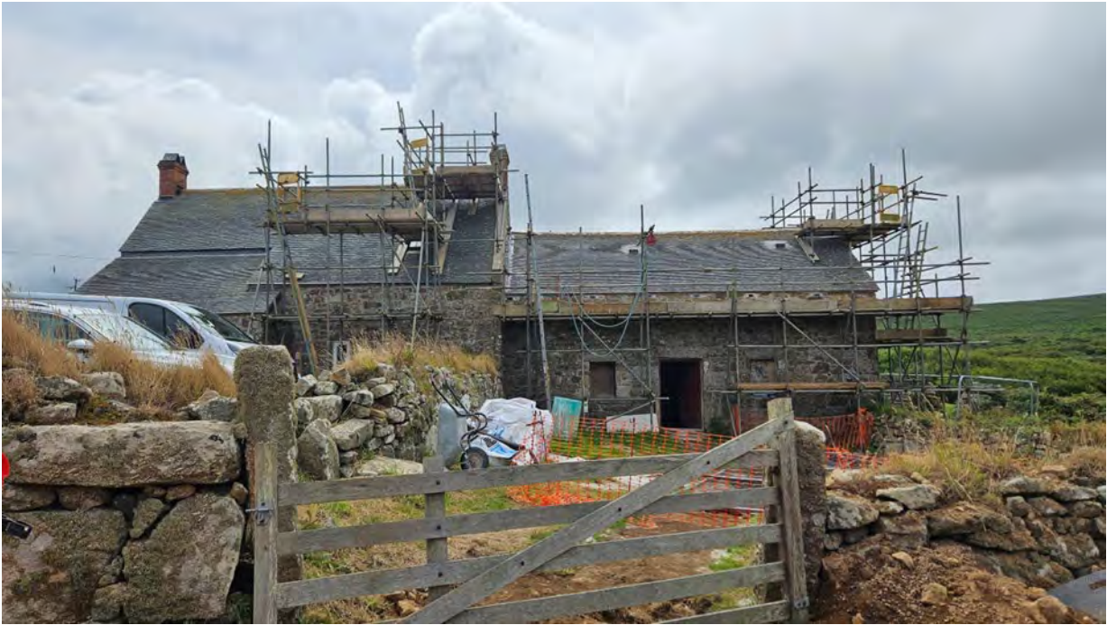
Work underway at Captain's House, summer 2025.
