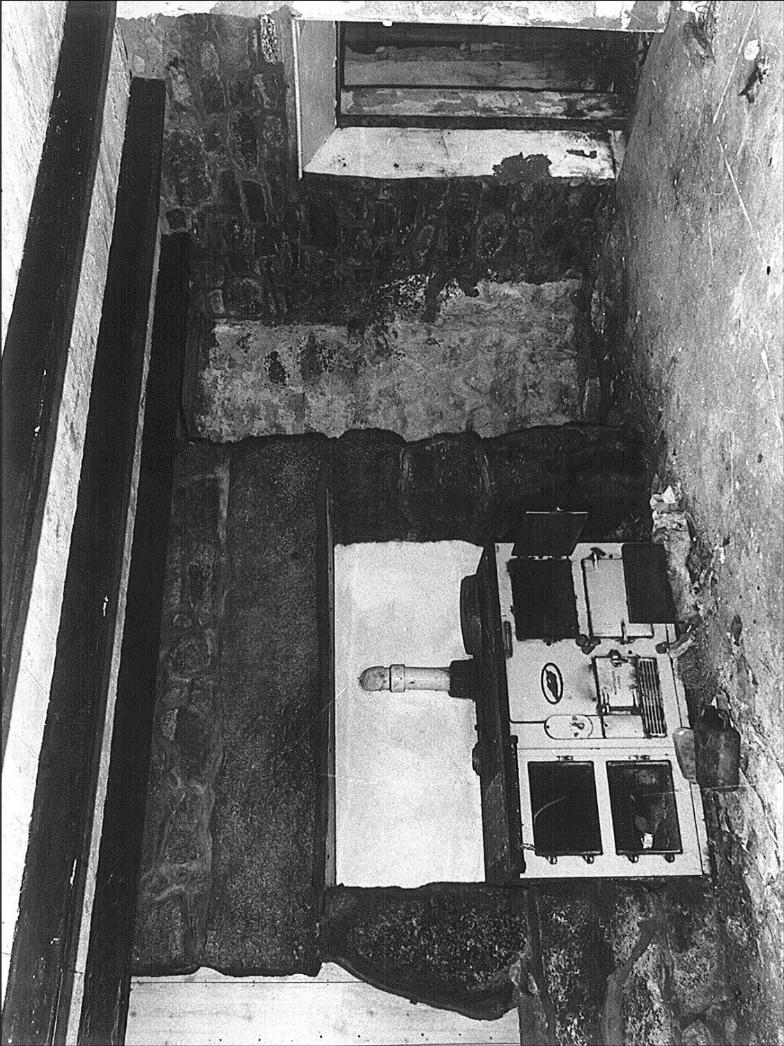
The Farmhouse: the great stone fireplace lintel is characteristic of many Penwith houses; this one has now been tamed with a wooden surround. The door into the dairy (more recently scullery)
