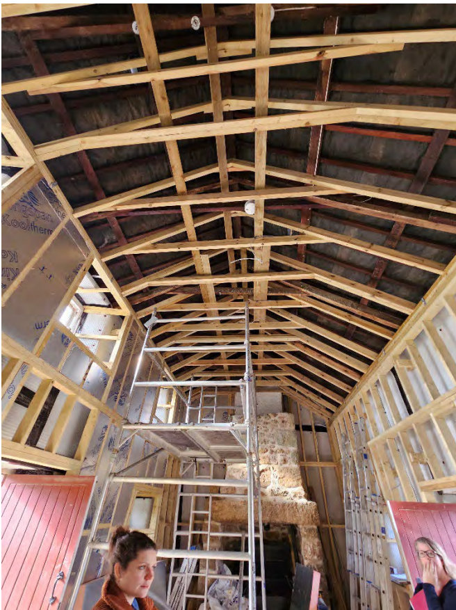
Once the barn had been cleared of its inserted boiler room, the massive cottage chimney breast was repointed and the walls lined out. An internal frame then was created to hang the ceiling from and to attach T&G panelling and insulation.
