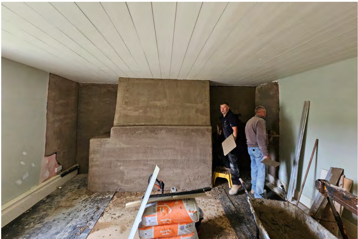
The Farmhouse first-floor west chimney breast under repair with insulation ready to receive lime plaster (below).
