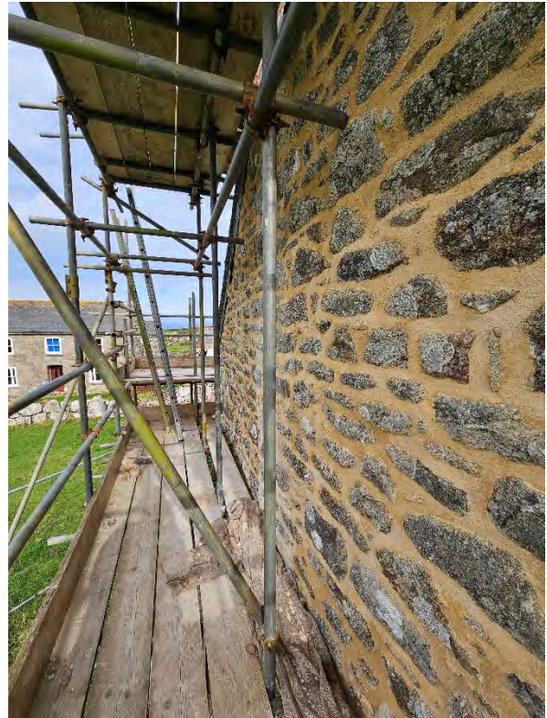
Repairs underway to the chimneys and scantle roof of Captain's House, and the repointed west wall of the barn end.
