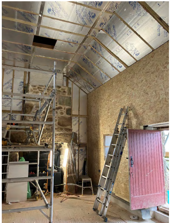
Once the barn had been cleared of its inserted boiler room, the massive cottage chimney breast was repointed and the walls lined out. An internal frame then was created to hang the ceiling from and to attach T&G panelling and insulation.
