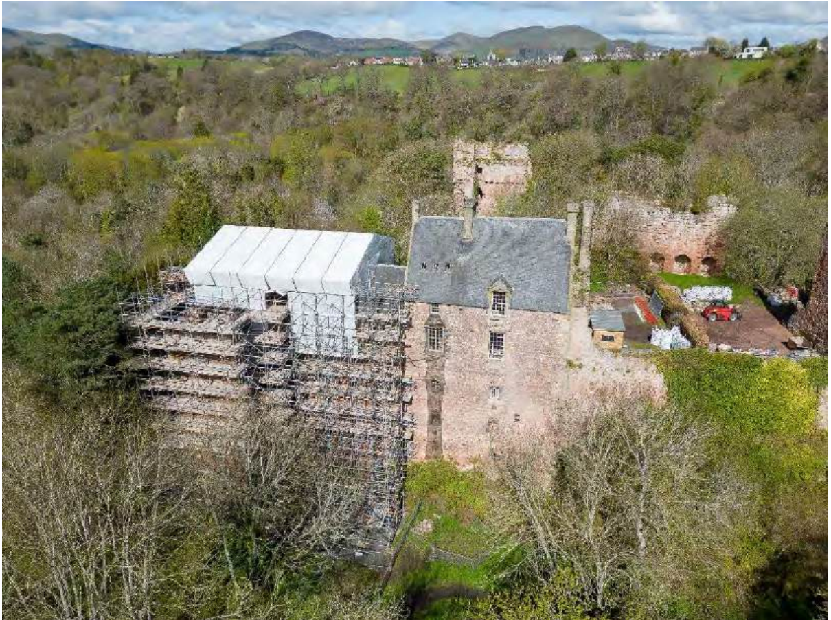
A canopy was installed, as part of the extensive scaffolding, to allow work to continue all year round (Picture: K Neville)
