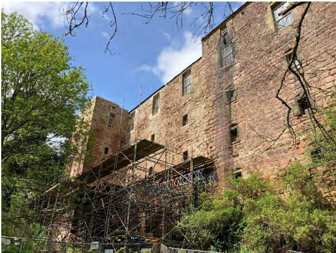
The stonework in the upper levels of the Castle was consolidated and repaired.
