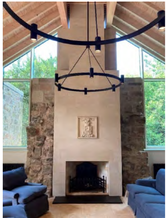
A new fireplace and chimney were installed in the west wall of the great hall, replacing a much earlier one.
