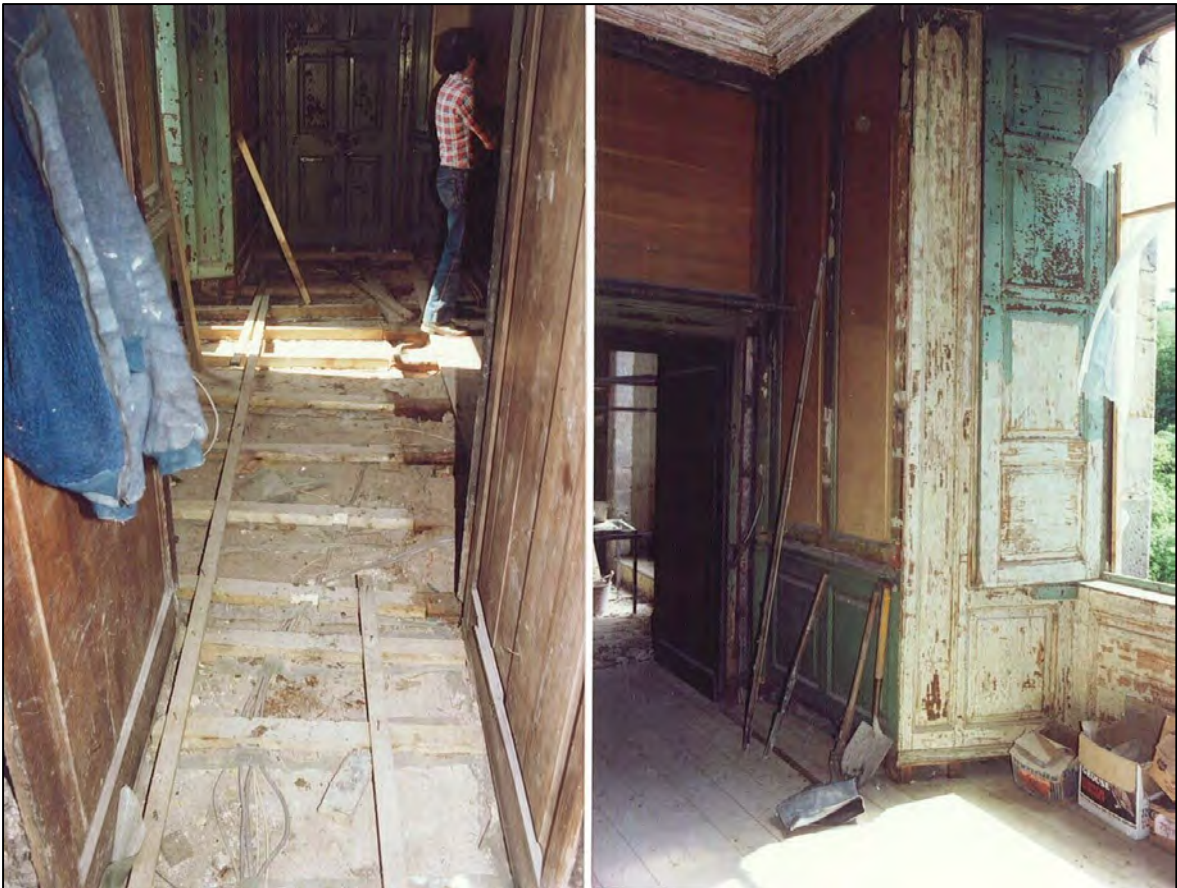
Repairing the panelling in the Dining Room, June 1984
