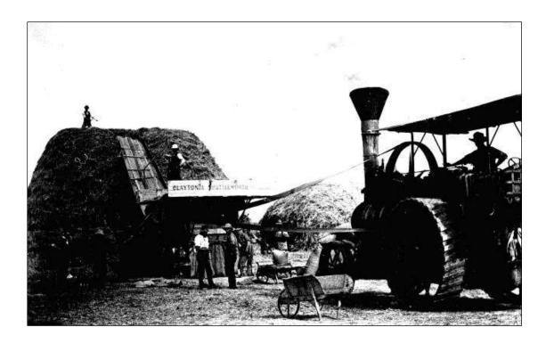
Clayton Shuttleworth threshers in operation in Australia at the turn of the century, powered by the traction engine.
