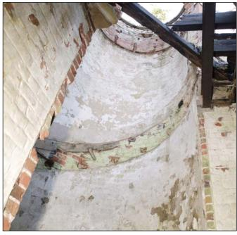
The main chamber was open to the sky through decaying rafters. The staircase timbers had collapsed into a pile in the basement, leaving only a paint scar and bearer sockets to show where it had formerly been.
