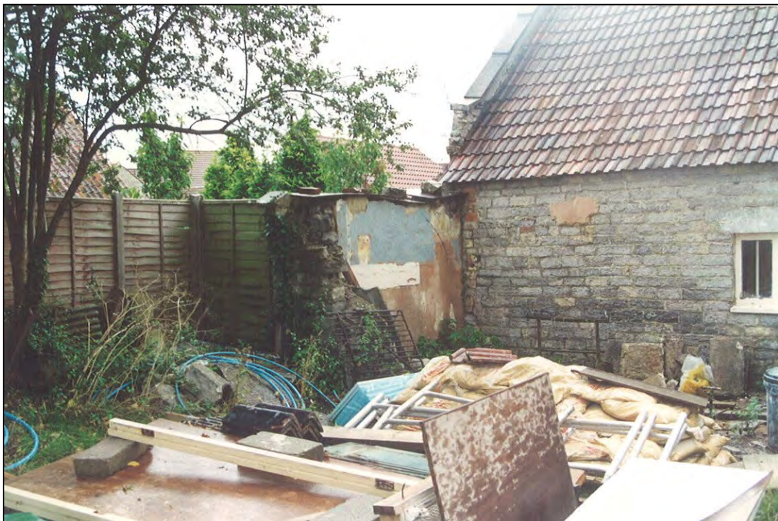
The roof was restored to its pre lean-to shape and the coping replaced.
