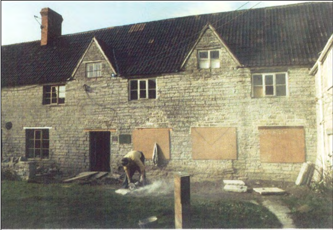
The windows on the ground and first floors were rotten and had to be replaced.
