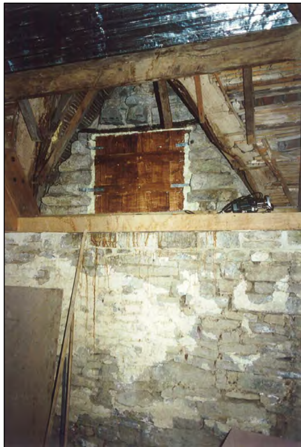
One of the blocked up dormers. The wall plate, damaged when the attic floor was put in, has been replaced.
