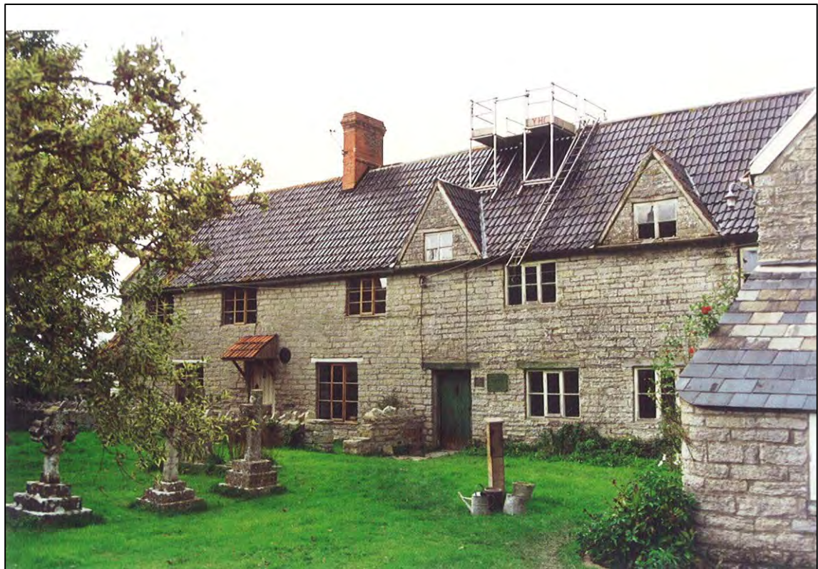
The central chimney, the low wall and the red tiled porch were all removed.
