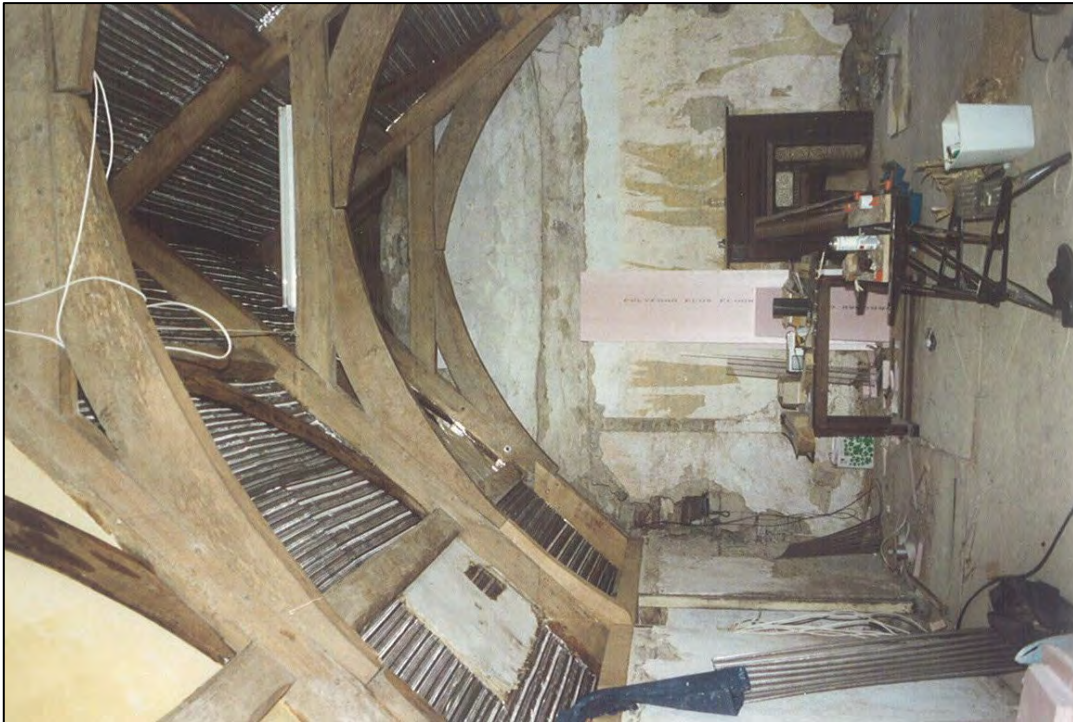
Looking east. Missing braces were restored, rotten and mutilated feet of the principal rafters were repaired and there were extensive repairs to the wall plates
