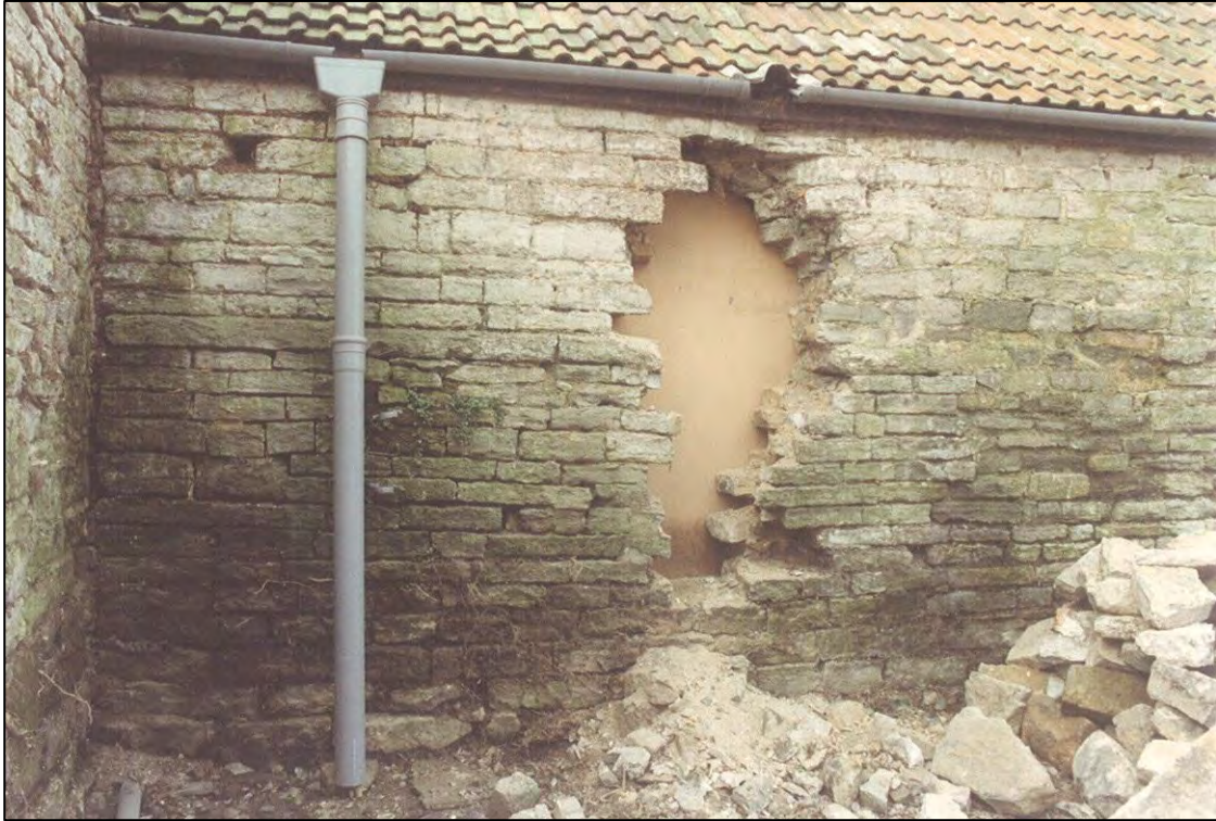
The opening for the front door.
