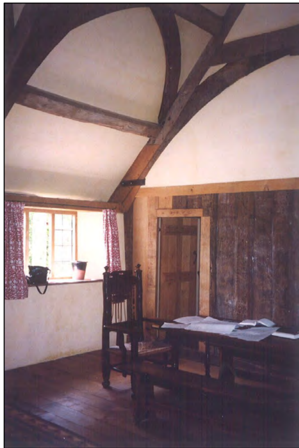
The repaired screen in its new position.
