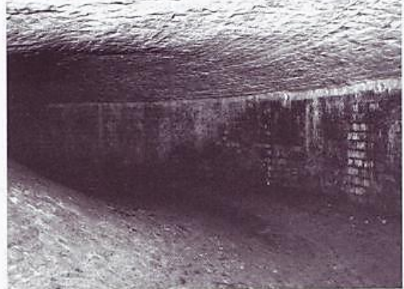
Empty water tank in base of Martello Tower 73. Base of rising central pillar at left (Andrew Goodwin)
