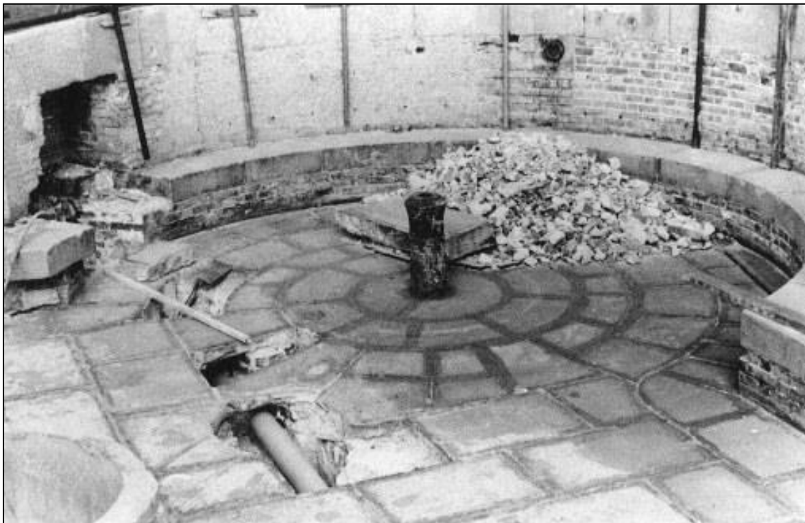
Work in progress on the roof. The pivot in the centre of the picture is an earlier cannon set into the roof when swivel guns were introduced. Above is an original restraining ring for the recoil chains of the gun carriage. To the left is one of the fireplaces of the 1930s
