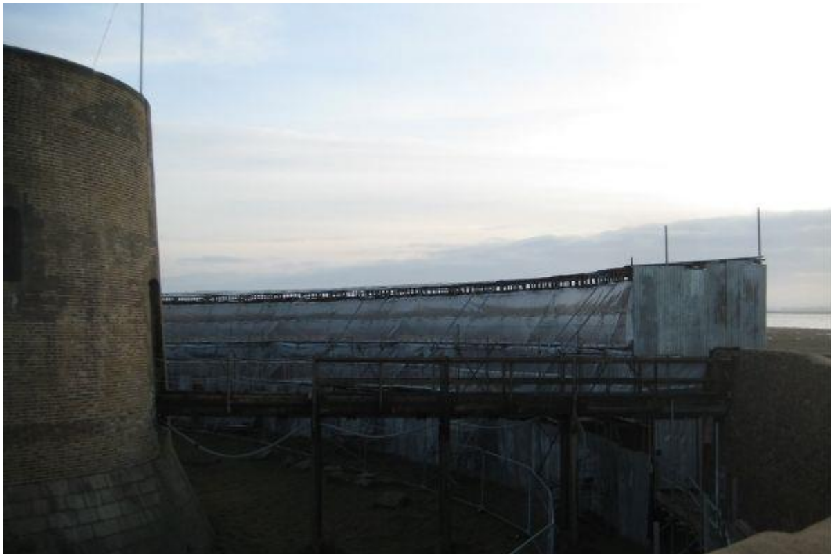
The glacis walls, scaffolded and sheeted against the elements for lime work in 2020-21.
