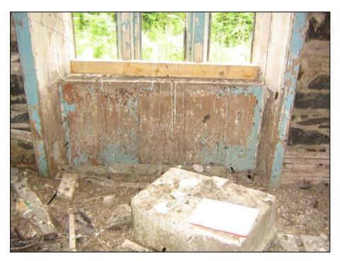
Fragments of surviving joinery before work began, on which the reinstated woodwork is based.
