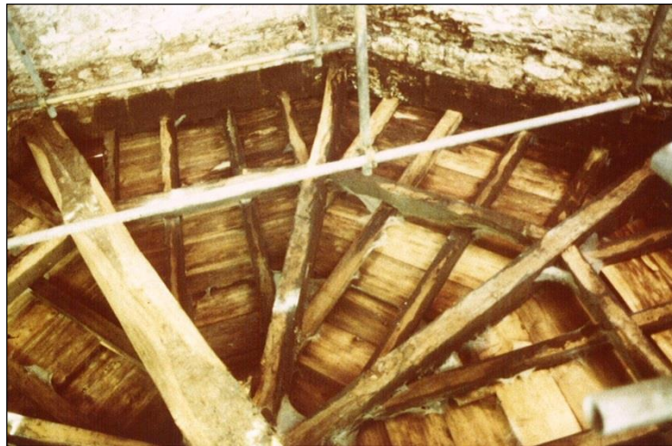
The roof structure exposed following removal of remaining plaster ceiling
