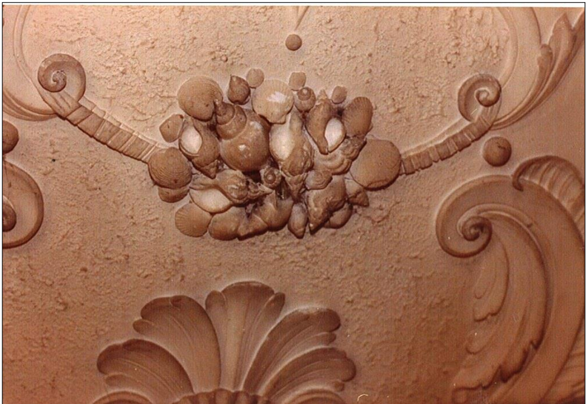
Original plasterwork salvaged from Upper Room ceiling before re-fixing
