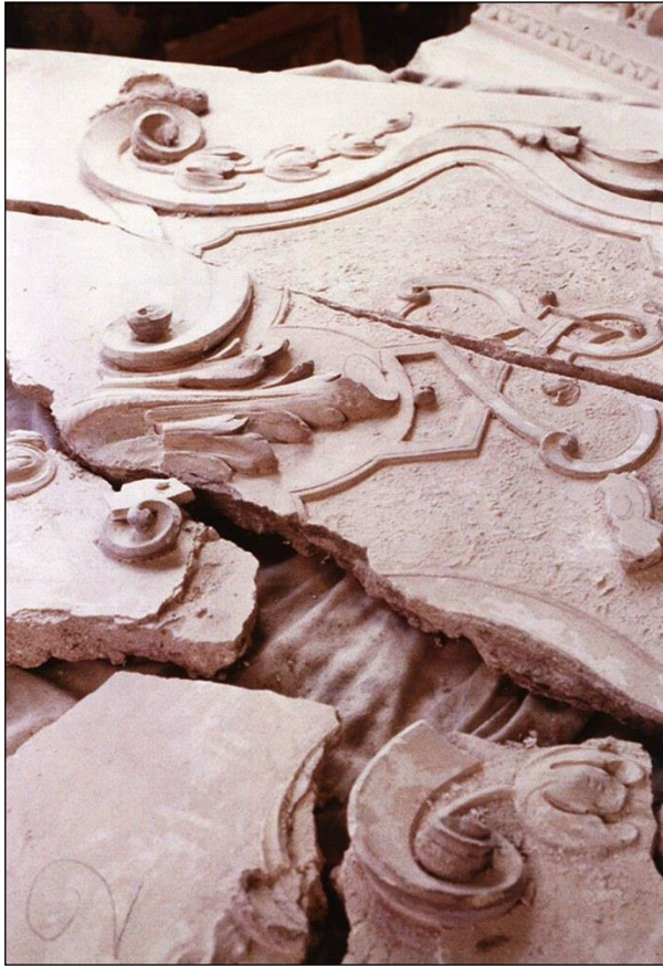
Original plasterwork salvaged from Upper Room ceiling before re-fixing
