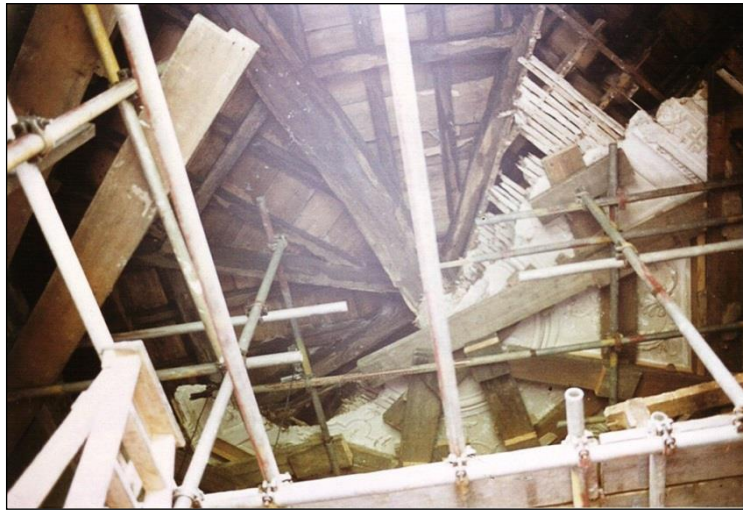
The existing ceiling propped
