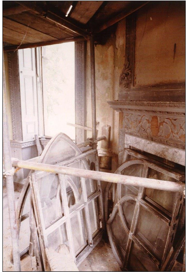
Joinery repairs in Upper Room
