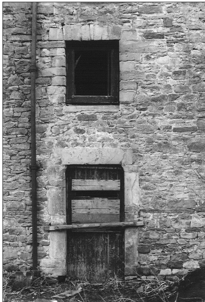
Door and window and North side, before
