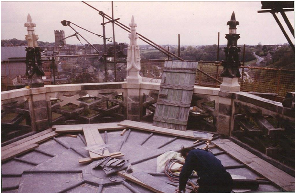
Completion of leadwork and stonework on roof
