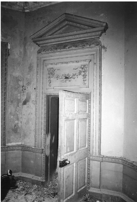
Doorcase in Upper Room, before
