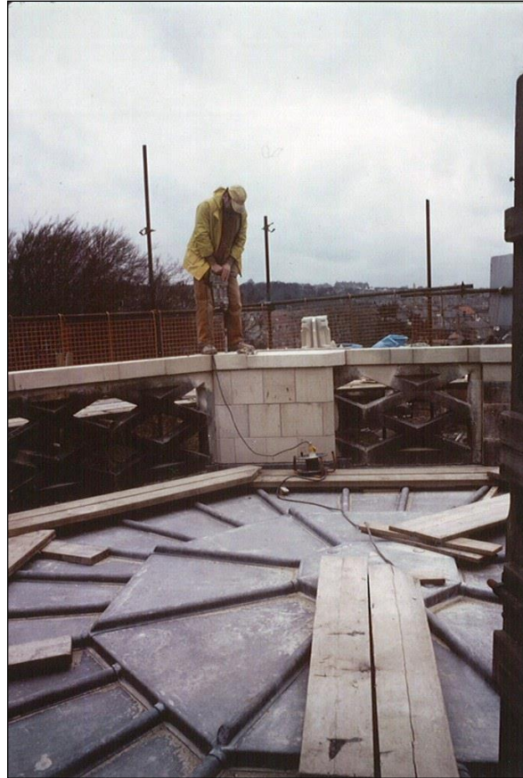
Inserting dowels for pinnacles
