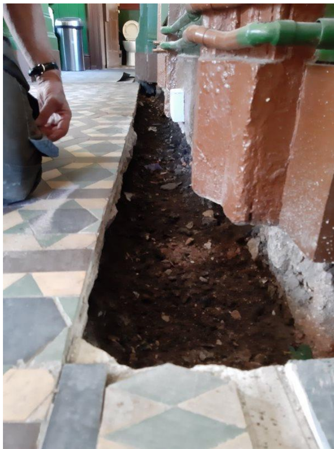
Burying unsightly pipework in the Waiting Room.
