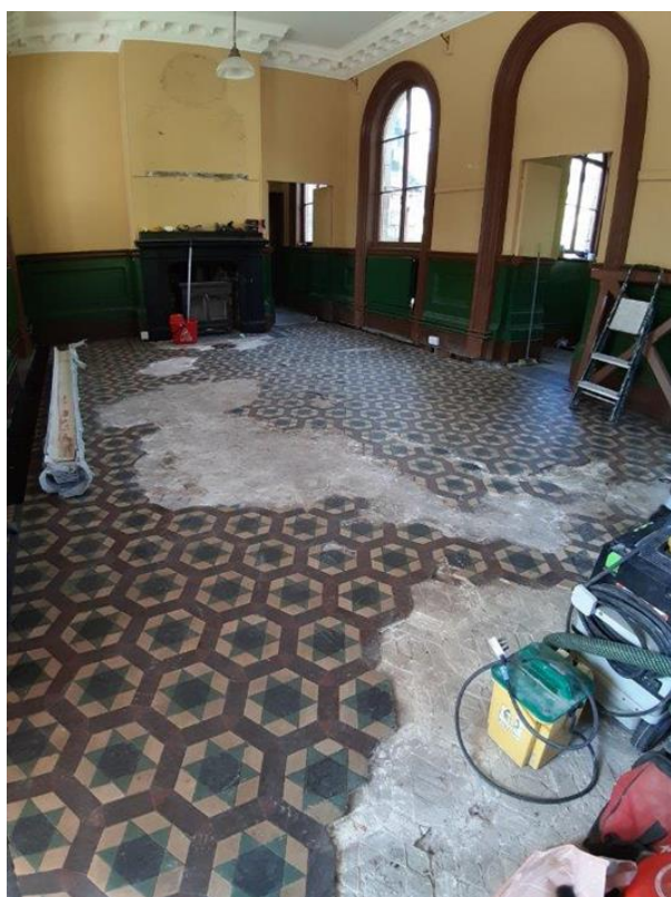
Left: Extent of the repairs, mirroring the areas of heaviest traffic in the past. Right: A group visit was organised for Landmark's Patrons to Winkhill Mill of Stoke on Trent to see the traditional production of dust-pressed tiles.
