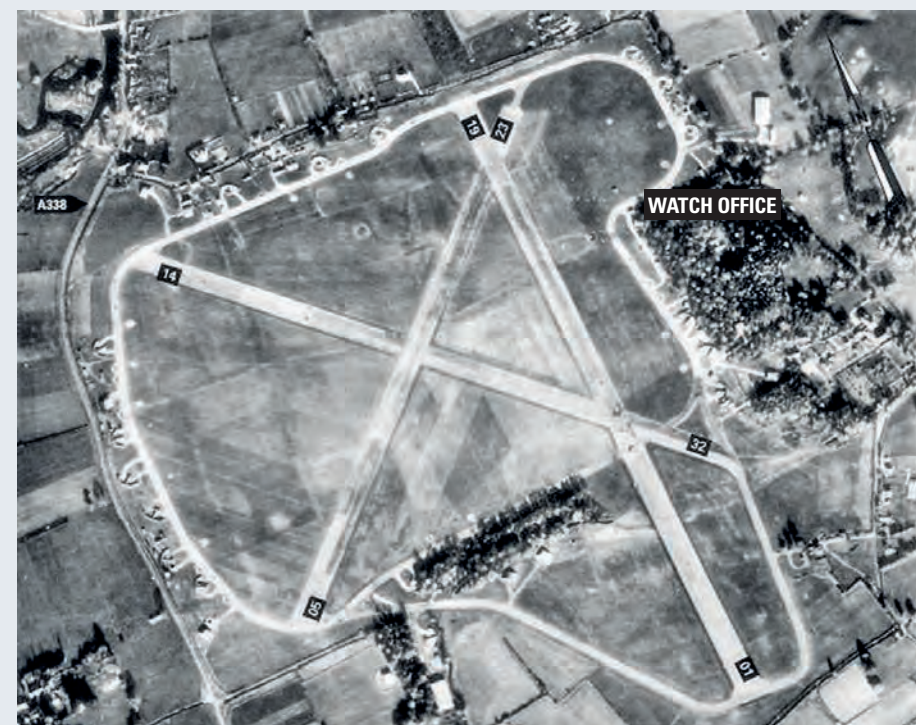
Aerial view of the runways at Ibsley, January 1944. The Watch Office is marked near the top right hand corner.
