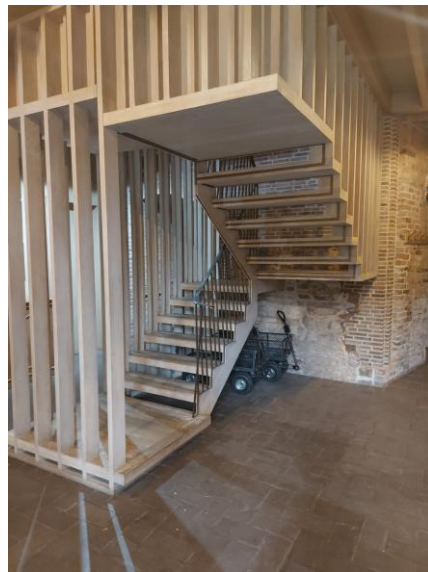
Stairs to first floor (each tread 18cm deep)
