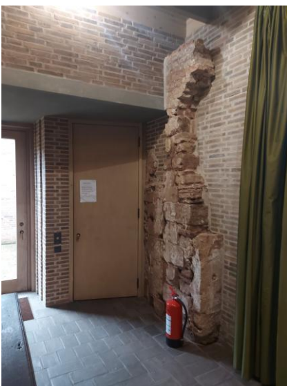
Lift door, on left in entrance hall
