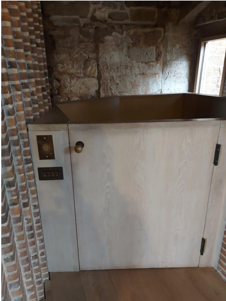
Lift door on first floor
