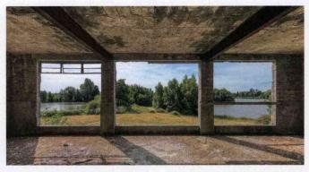
concrete viewing balcony and the Meteorological Section, where the Women's Auxiliary Air Force collected vital data on weather. However, the structure's large Crittall windows have rusted and fallen in and the ceilings are rapidly collapsing. According to the Airfield Research Group, it is among the best most-at-risk of buildings of its type.
