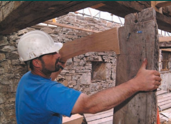
Above To restore the roof, a 40-foot crane arrived on site to lift the three massive roof trusses back into place. A craftsman pieces together Dolbelydr's internal timber frame.
