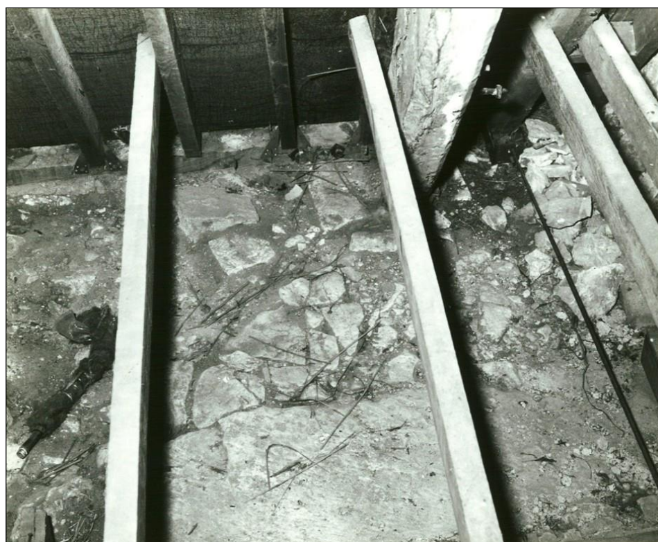
The smooth surface of the medieval wall walk, still visible on the wall head
