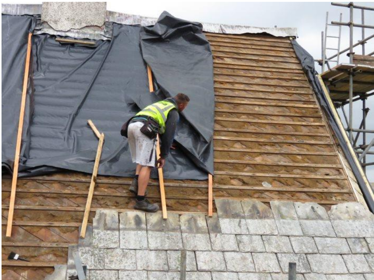
The day room has been taken down. Note the fire escape door, now returned with its fellow opposite to windows. Below: stripping the Delabole slate roof. The original sarking boards, battens and horsehair insulation survived but were leaking.
