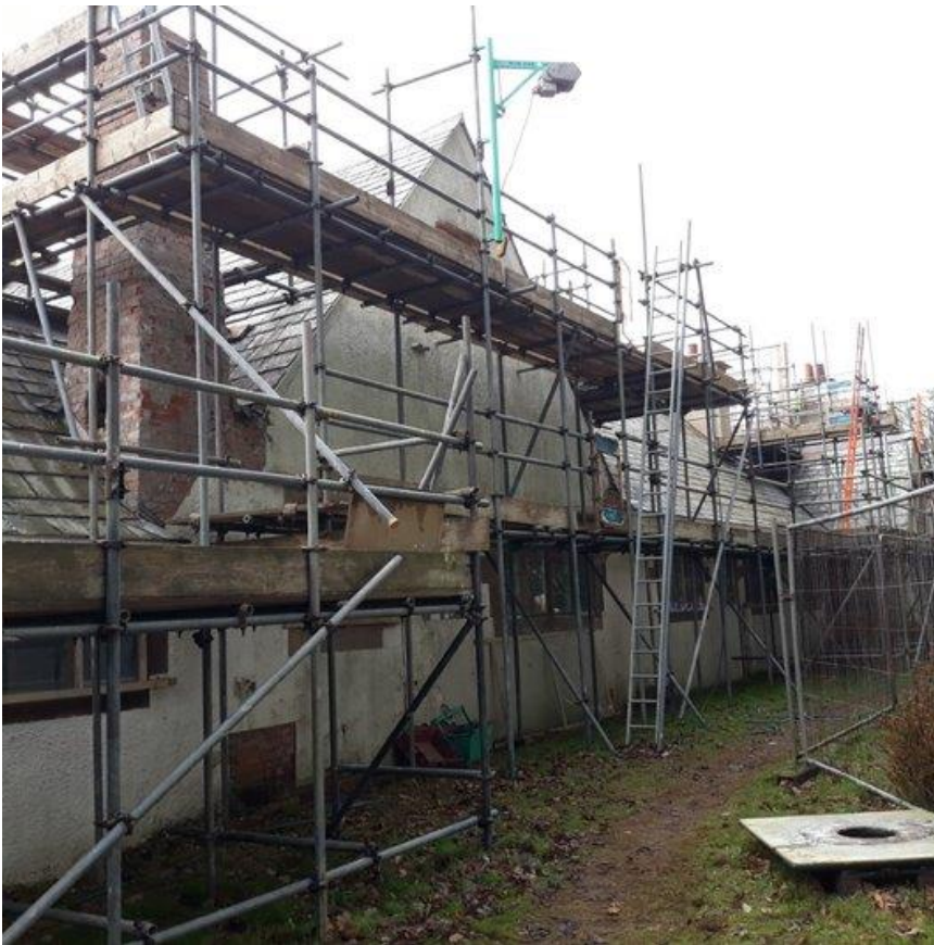
The building was entirely scaffolded as work got underway in autumn 2018.
