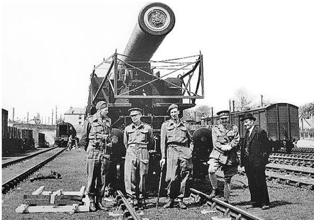
Top: Looking north from Halwill Junction in the 1930s. Below: The sidings during WW2: a Howitzer railway gun in 1944 The eight wartime sidings must have made the hospital very noisy.
