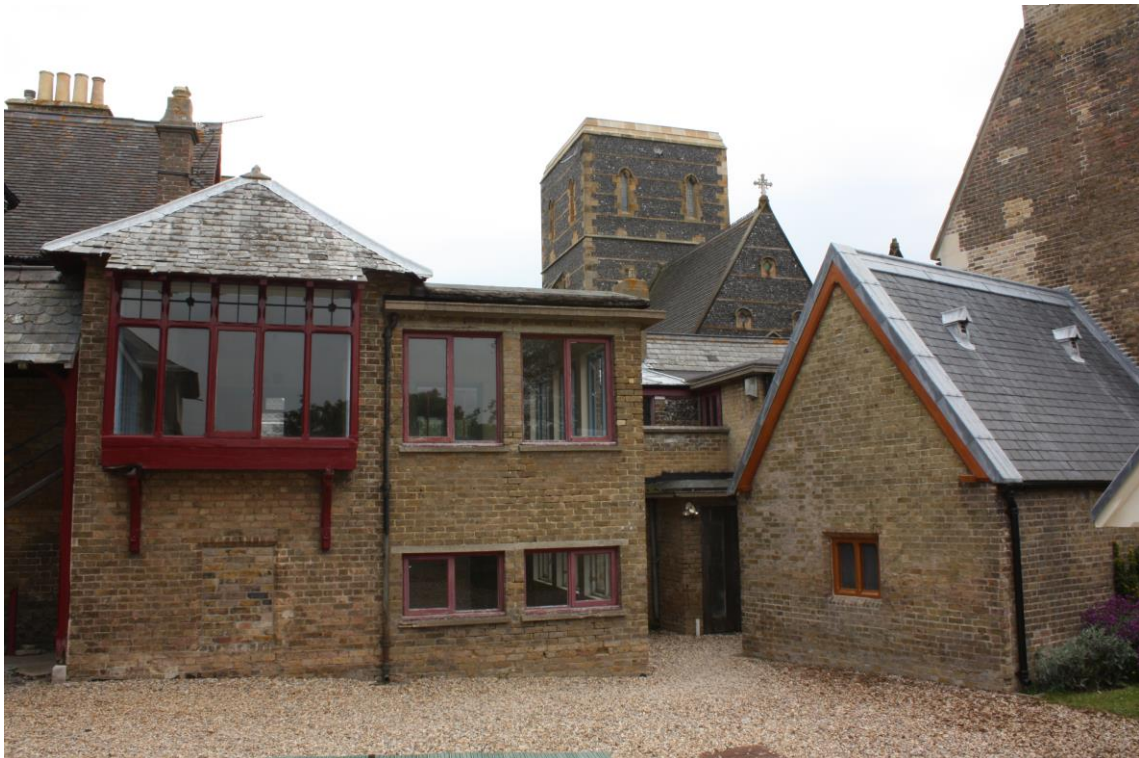
Looking east in the north courtyard, the 20 th -century classroom extensions have engulfed Edward's studio.
