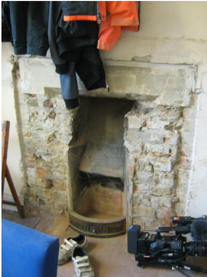
Unpicking the original opening to the kitchen hearth.
