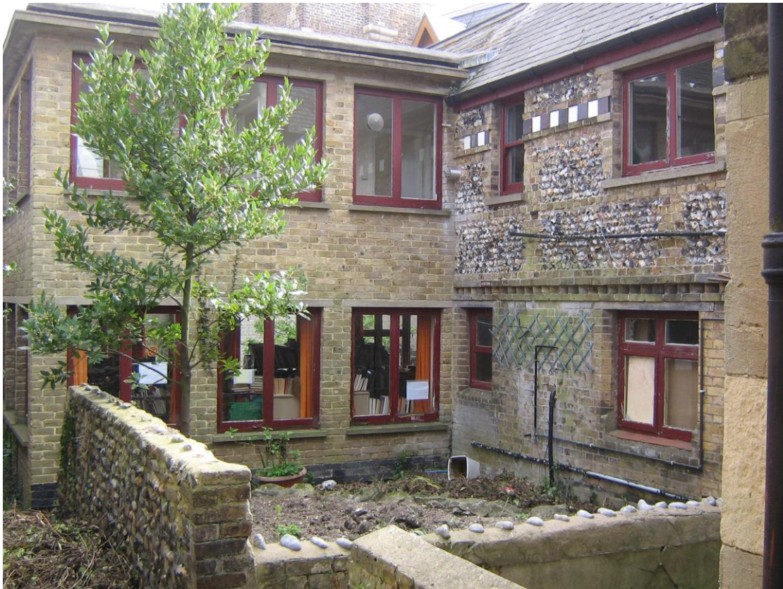
The view from the back door of The Presbytery before restoration.
