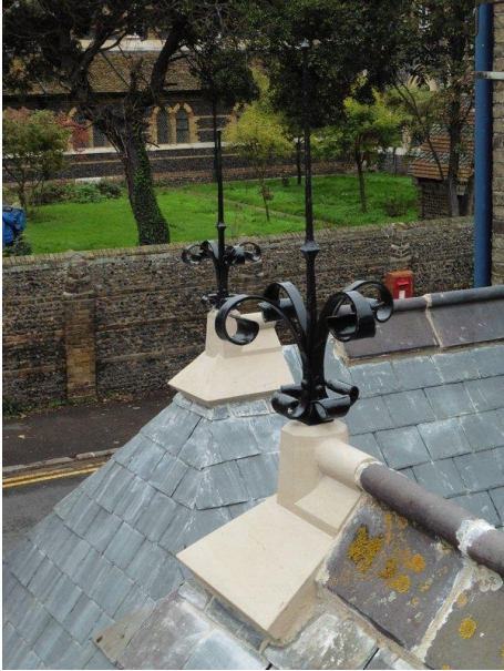
The re-made finials are steel, hot-dipped and galvanised against corrosion, made by blacksmith Bob Oakes
