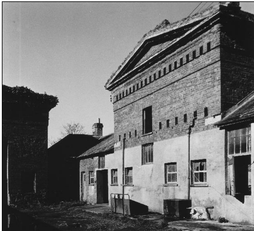
The courtyard face of the north range before work began.
