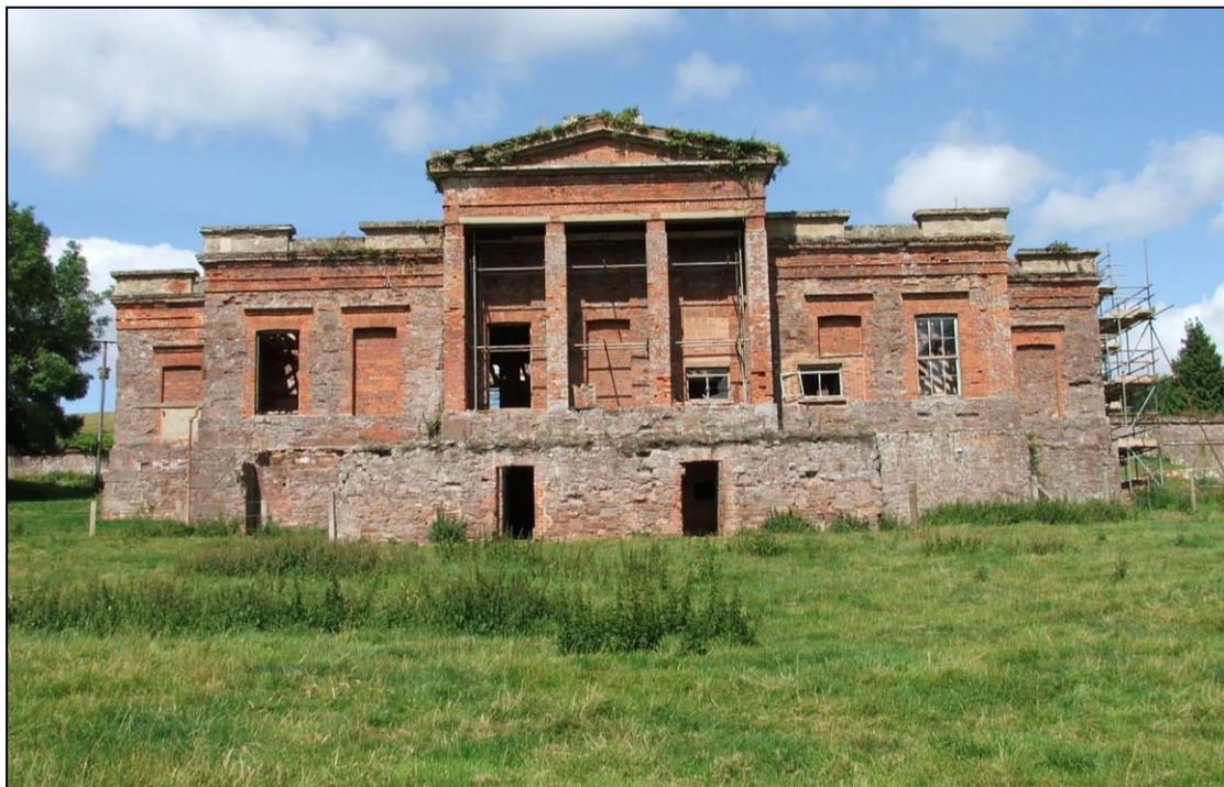
The south elevation before work began.
