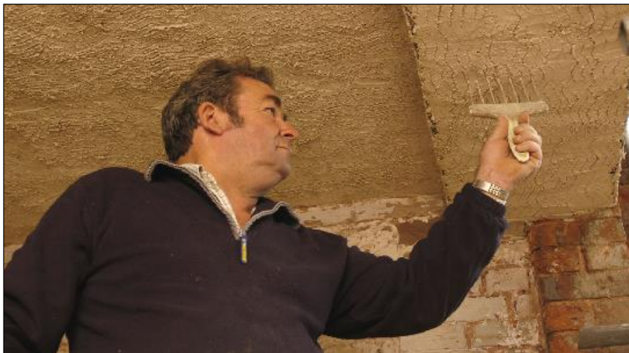
Putting on the scratch coat for a ceiling.
