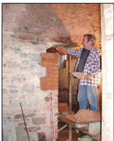
Repairing decayed brickwork in the southwest corner, Nov 2005
