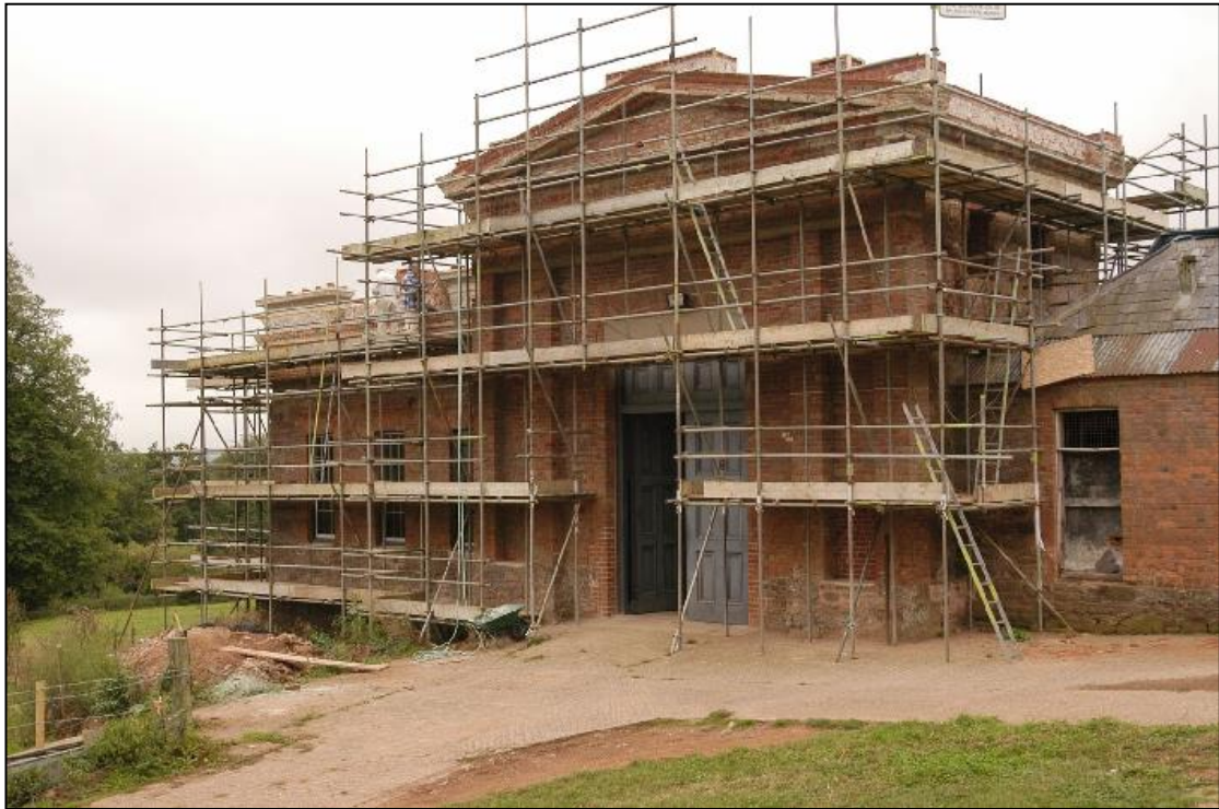
The east elevation scaffolded, with work going on to the cornice.
