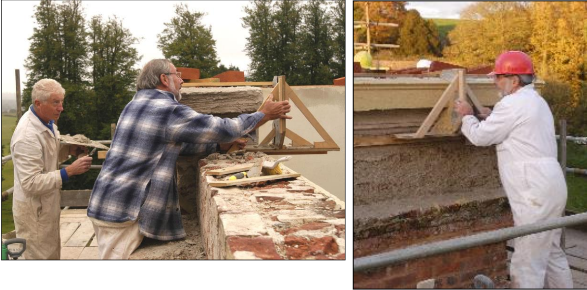
Alan and Stan Flood running in the parapet cornice. The former used is known as a 'horse'.
