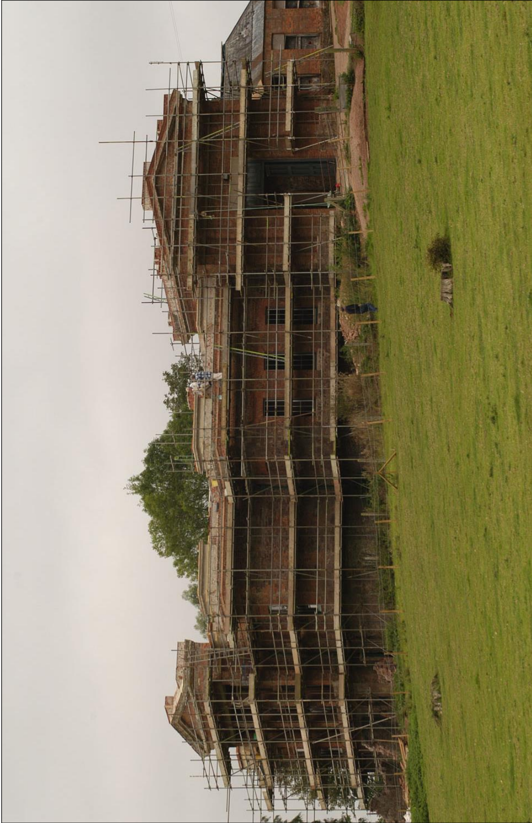
The stable block in October 2006, fully scaffolded.
