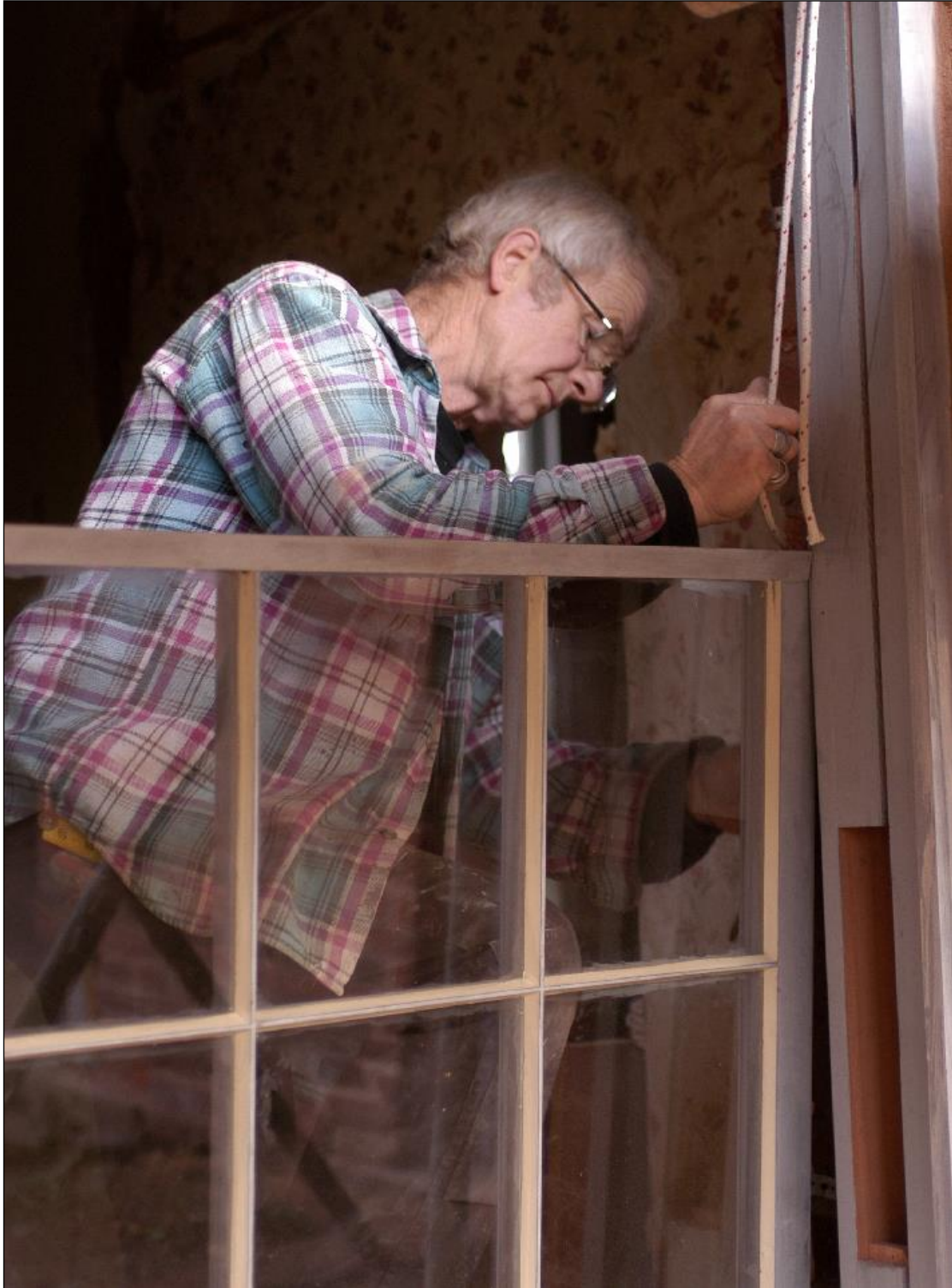
Fitting new sash cords is a fiddly business unless you know the system.
