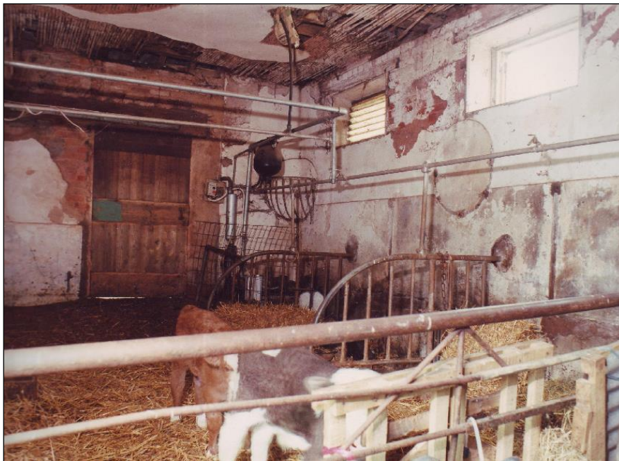
Interior of the east range when in farm use.
