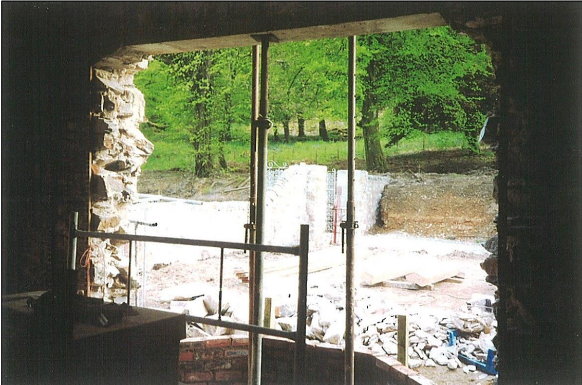
The new window bay
