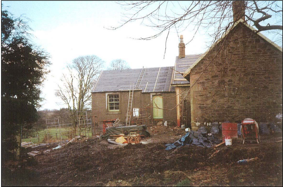
Work underway in 1985 on the roof and extension.
