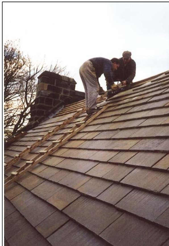
Fixing the last of the stone slates to the roof
