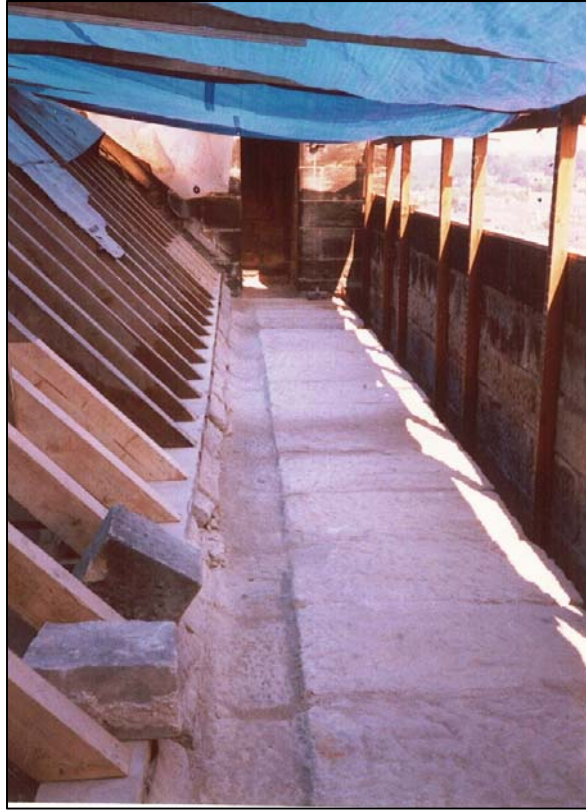
Open day, summer 1990, with roof stripped
