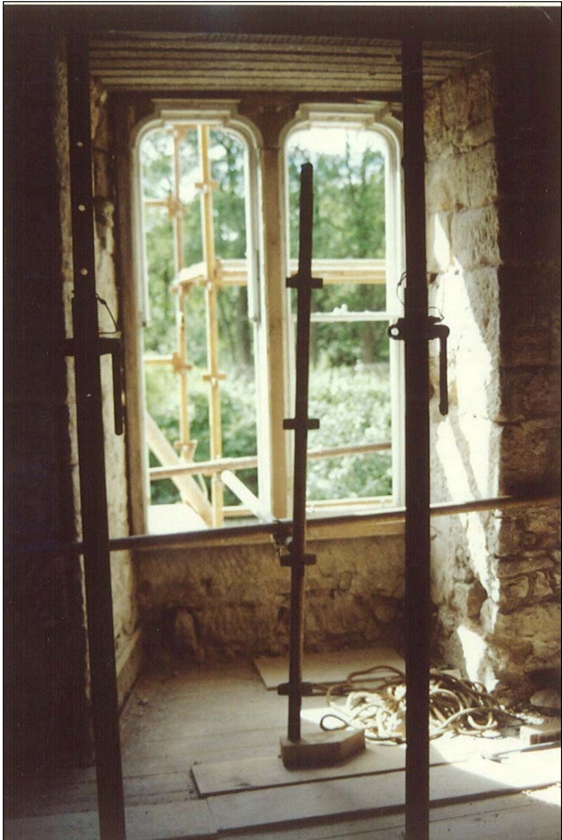
Window onto the second floor passage. The level of the original floor is shown by gaps in the stone work.
