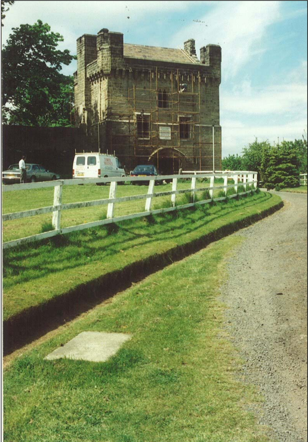
The last of the scaffolding coming down.
