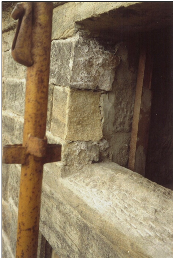
Finding the 17 th -century windows in the attic.
