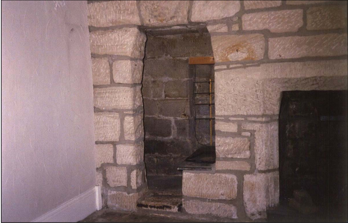
Opening made in 1960s into garderobe on north end of first floor, now built up.
