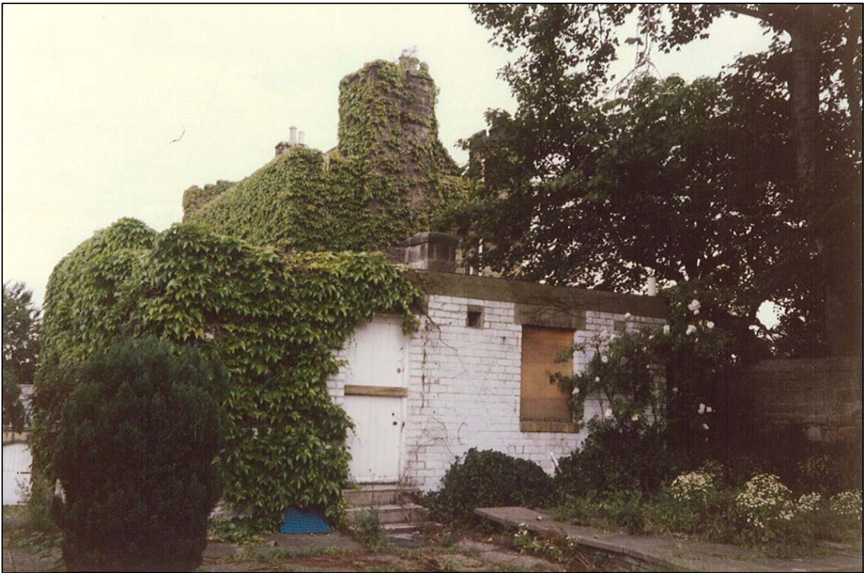
The south side with extension in 1986
