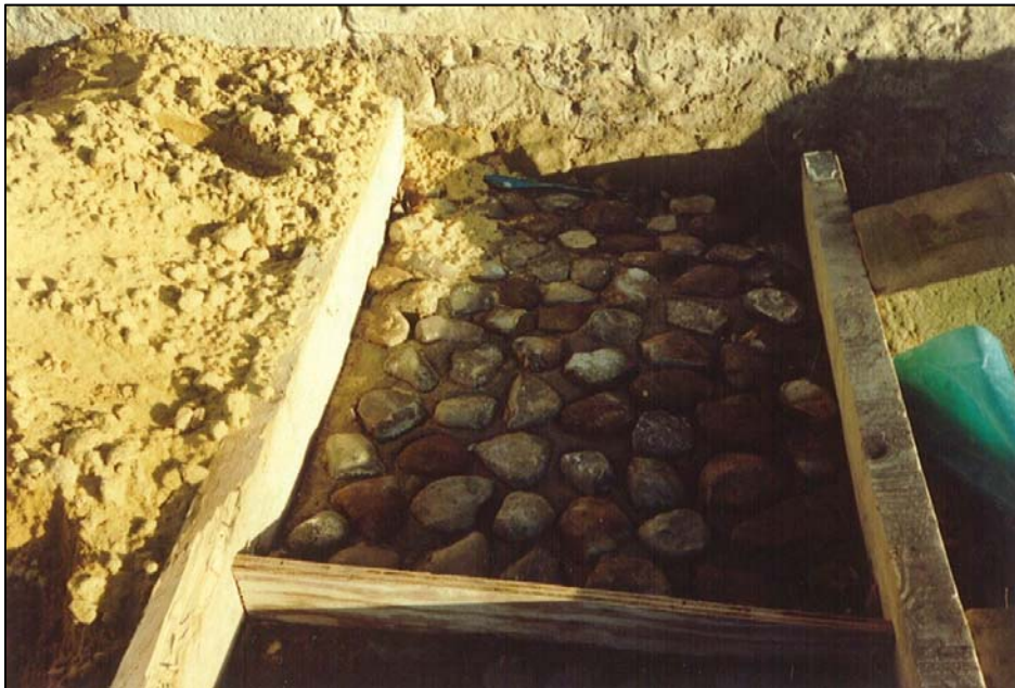
Practising laying a cobble pattern
