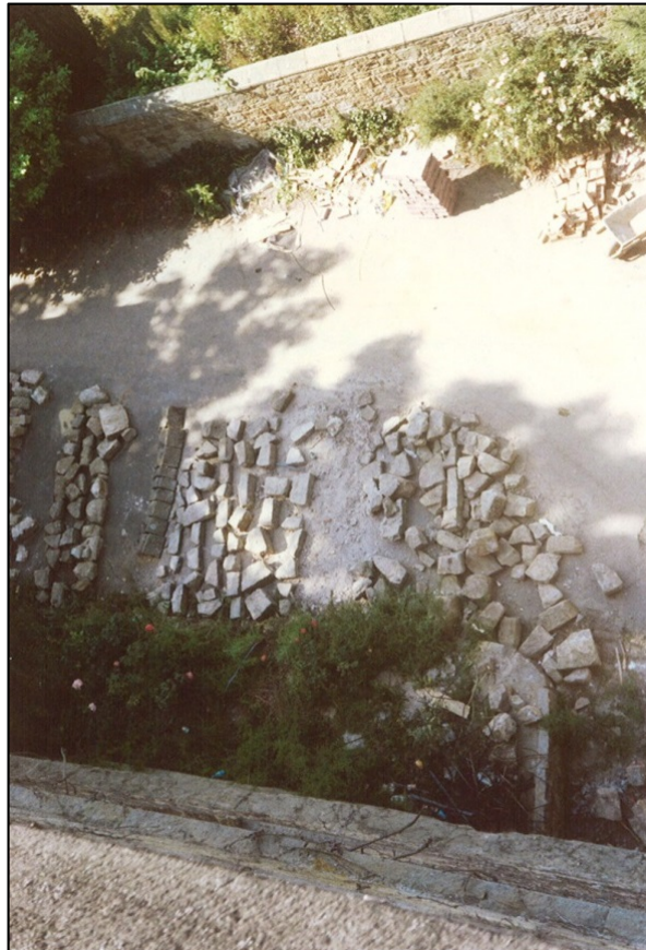
The sets laid out before being put into position
