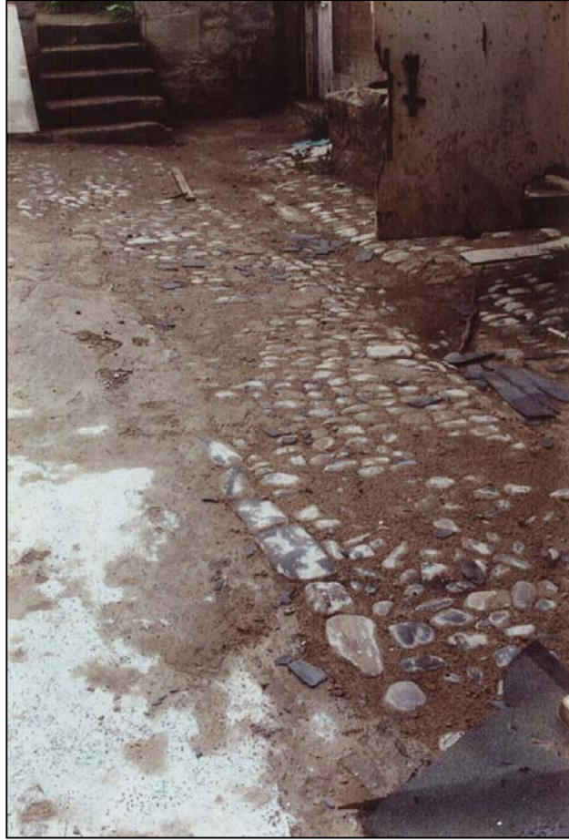
Outside the stables showing original cobbles
