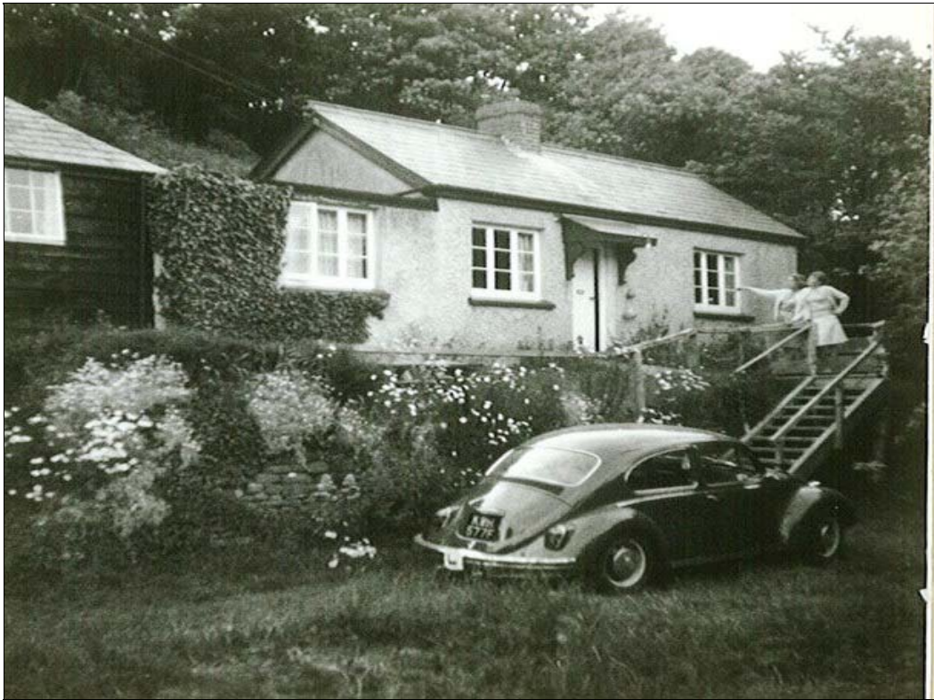
Chapel Cottage before restoration
