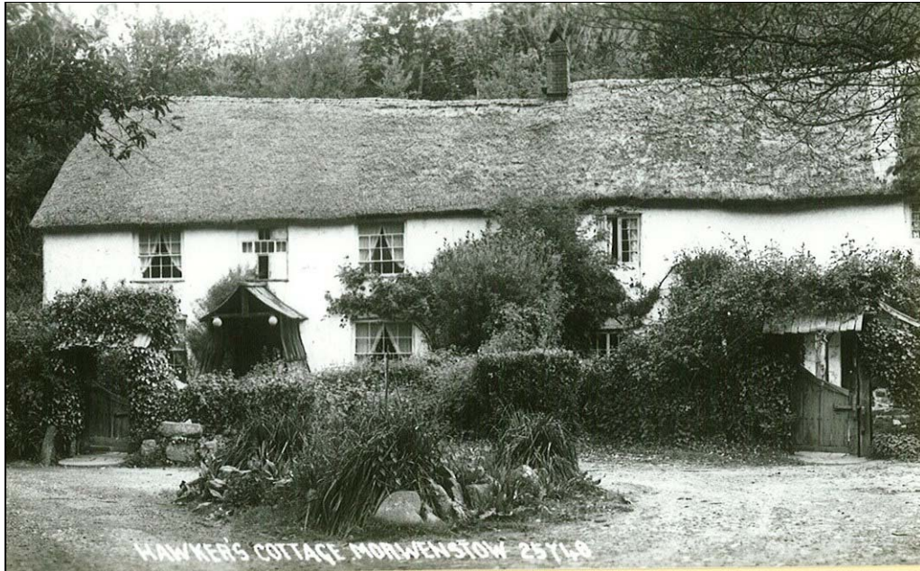
Hawker's cottage before restoration
