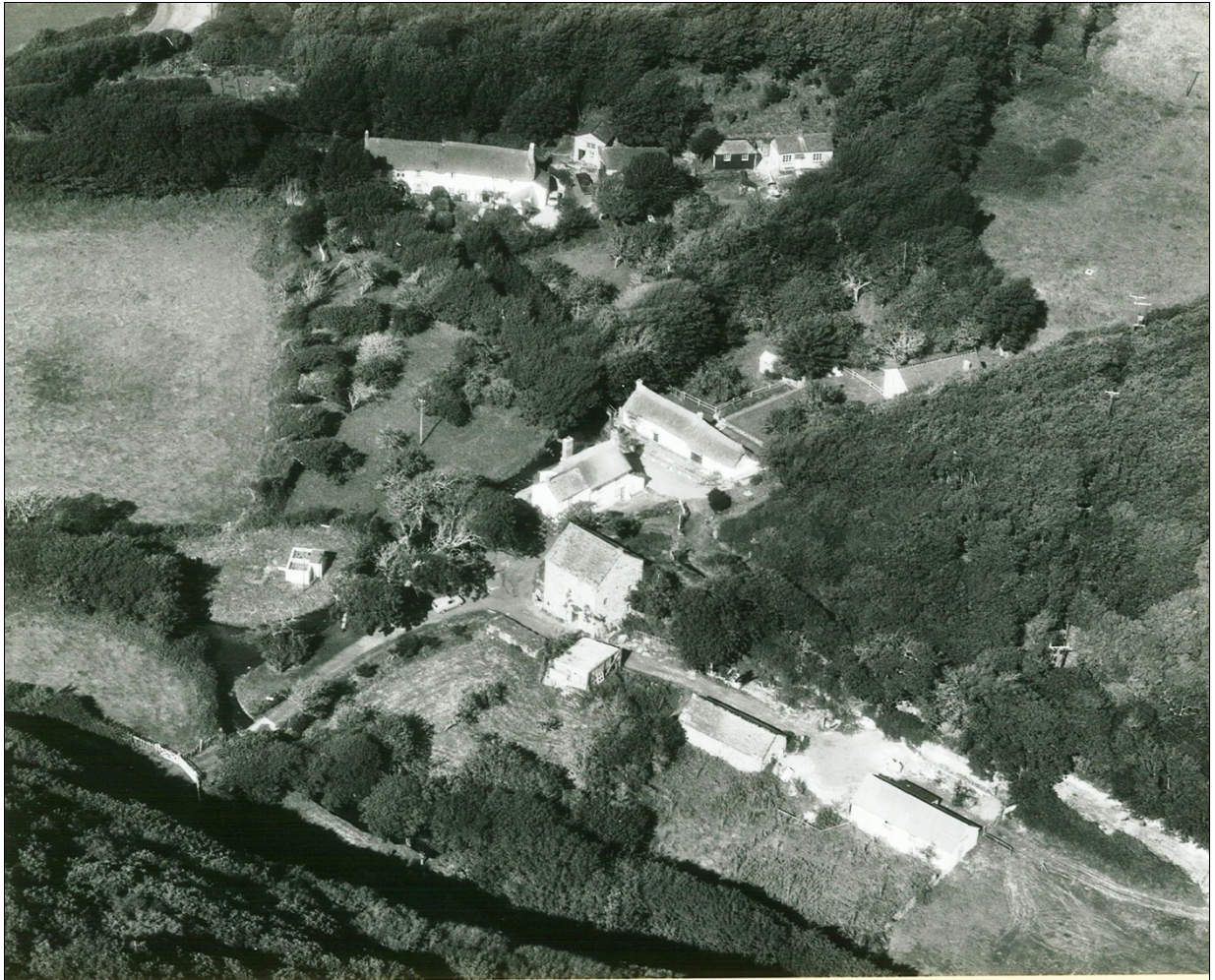
Coombe in 1969 when Landmark's repairs were in progress. The Mill House, Ford Cottage and the Carpenter's Shop are complete, work is underway on Chapel Cottage.
