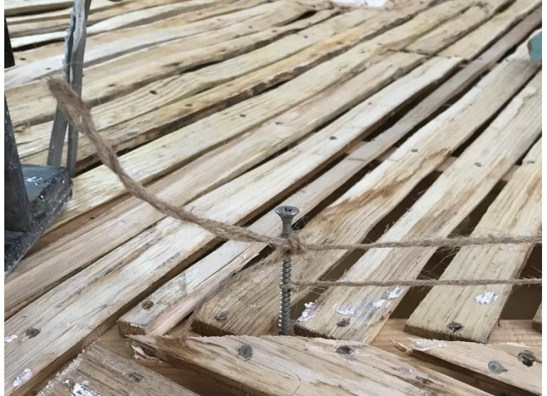
Creating the plaster ribs: the patterns for the profile; string is used to reinforce the line; all ceilings and walls had to be re-lathed, and Anna Castilla Vila working on the ribs in the south cloister (today's kitchen, the end doorway boarded up for protection during the works).
