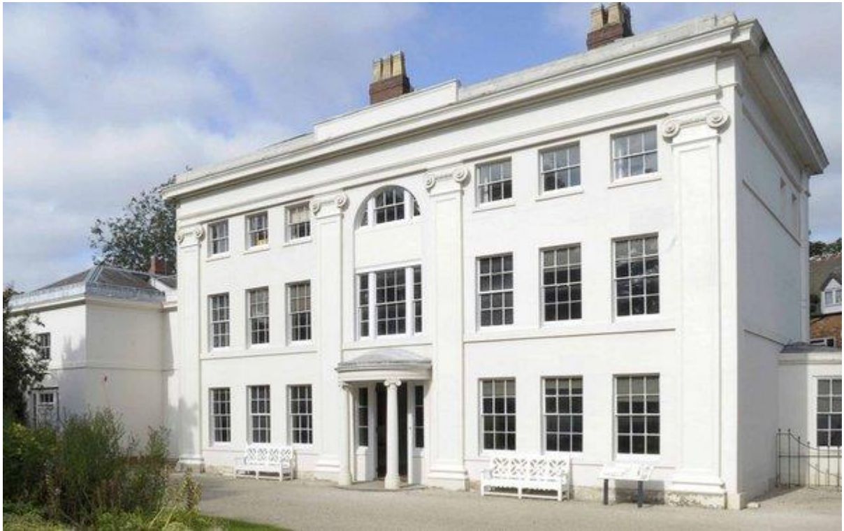
Soho House, Handsworth, Birmingham. Industrialist Matthew Boulton's former house, both James and Samuel Wyatt worked on adaptations here. This south elevation is still entirely faced in original slate cladding identical to that used at Cobham Dairy.
