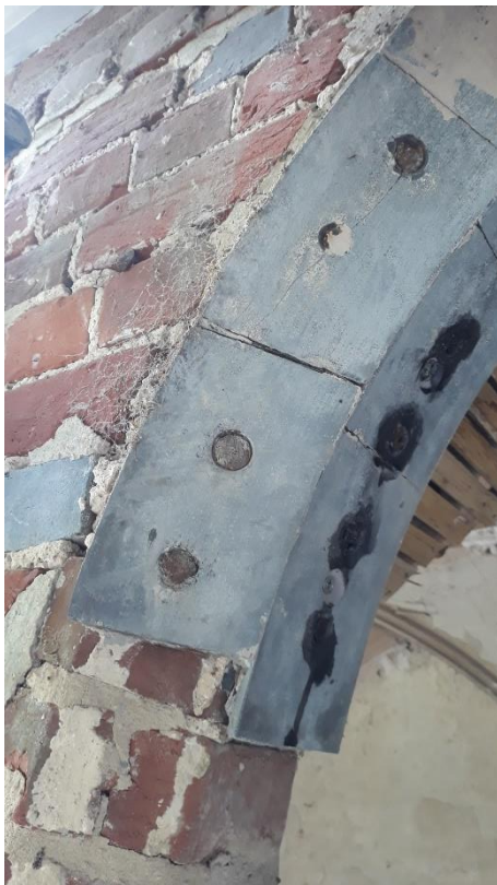
The original slate cladding on the west gable was still sound, and skilfully shaped fragments also remained in some of the cloister openings. There were enough usable salvaged slates for the upper, clerestory level.
