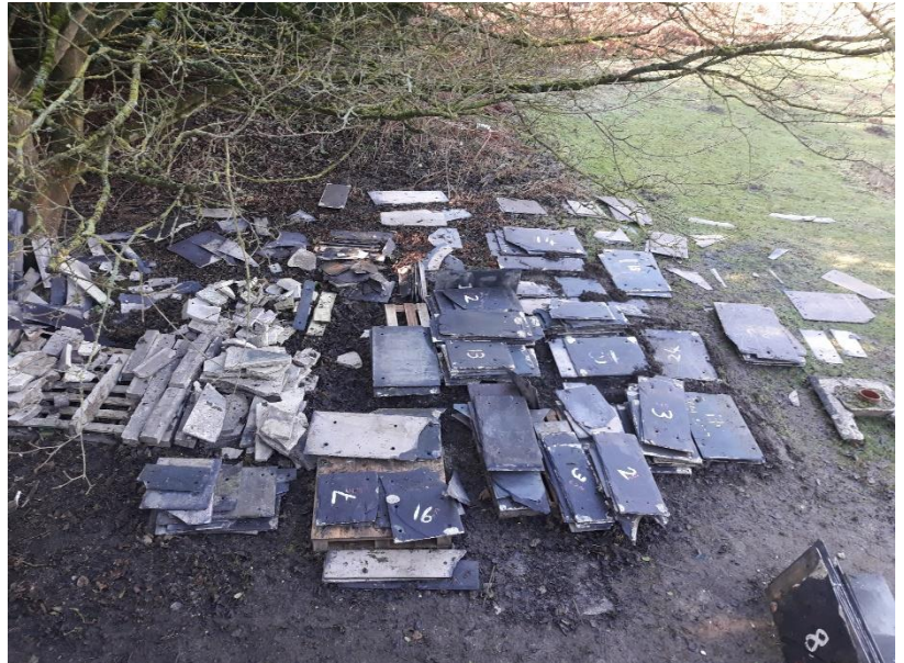
The original slate cladding on the west gable was still sound, and skilfully shaped fragments also remained in some of the cloister openings. There were enough usable salvaged slates for the upper, clerestory level.
