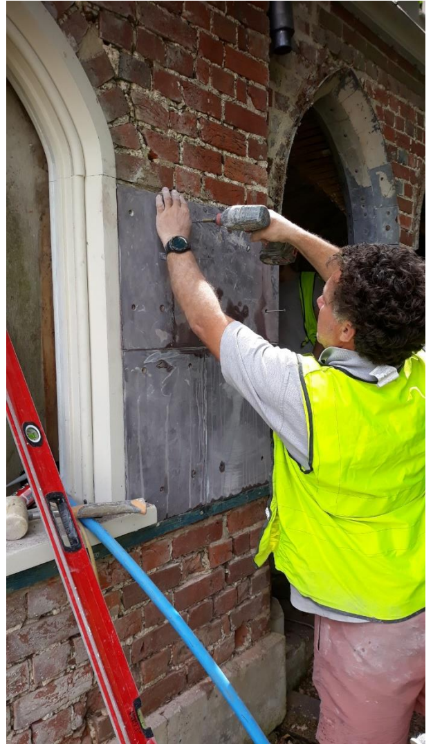
Repairing the slate cladding. A lime mortar bedding allowed a flush surface to be achieved, before fixing the slates with stainless steel nails into the brickwork joints – an exacting task, especially around the openings.
