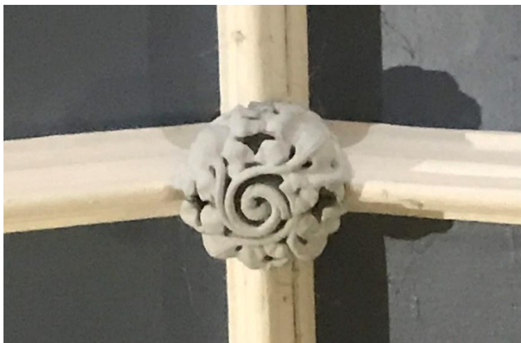
Examples of Francis Bernasconi's work for Wyatt in Cobham Hall (entrance lobby). Note too the glass screen with coloured slips and painted bearings.
