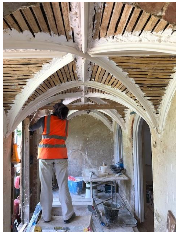
Creating the plaster ribs: the patterns for the profile; string is used to reinforce the line; all ceilings and walls had to be re-lathed, and Anna Castilla Vila working on the ribs in the south cloister (today's kitchen, the end doorway boarded up for protection during the works).
