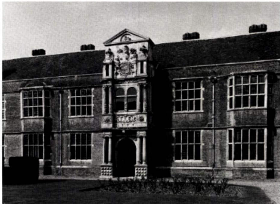
4—THE PORCH ON THE SOUTH SIDE OF THE NORTH WING. Dated 1594, it was probably re-erected in the early 1660s and altered in the late 1760s
