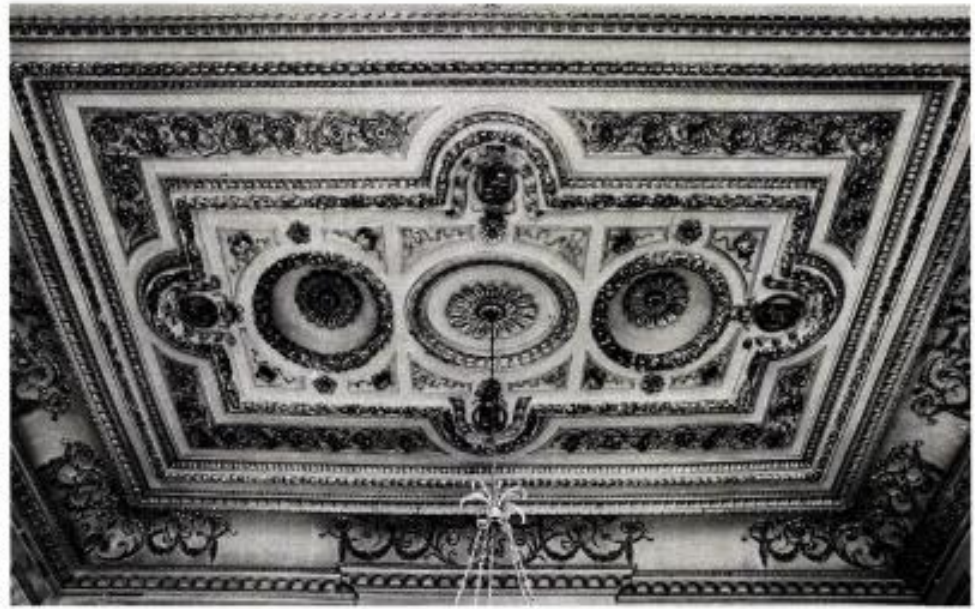
8—THE CEILING OF THE GILT HALL. The plasterwork was ready for painting in 1672; and some additional ornament was added about 1770
