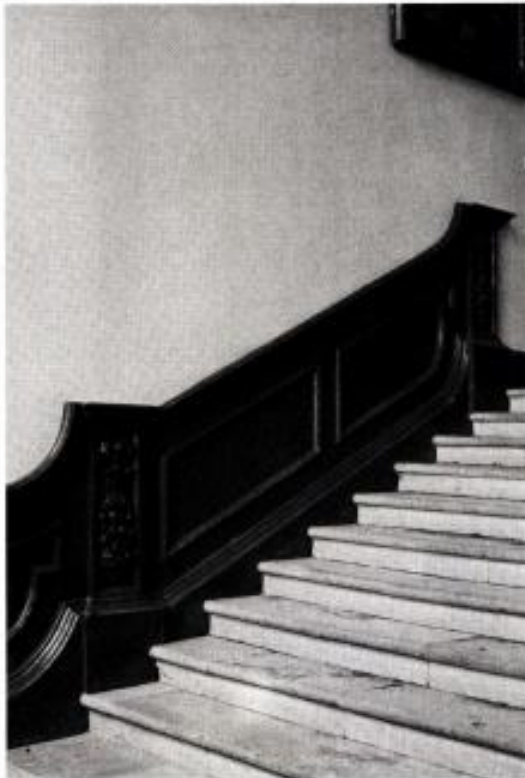
9—A DETAIL OF THE STONE STAIRCASE. A section of the Restoration woodwork
