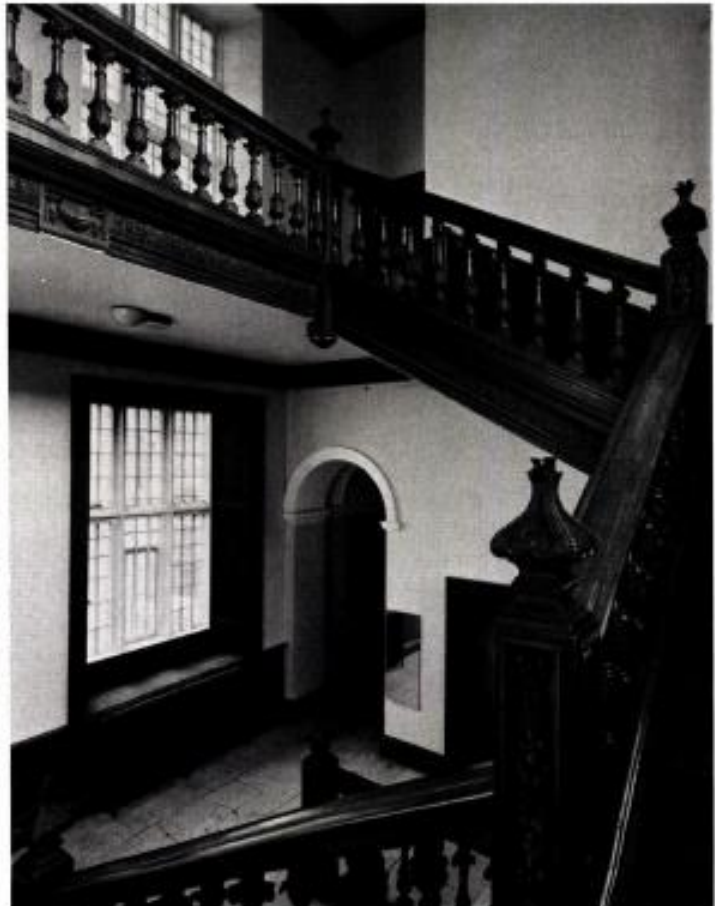
(Right) 10—THE OAK STAIRCASE. The balustrade dates from the 6th Duke's time but it is not in situ
