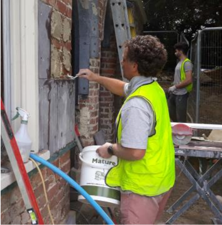
Repairing the slate cladding. A lime mortar bedding allowed a flush surface to be achieved, before fixing the slates with stainless steel nails into the brickwork joints – an exacting task, especially around the openings.
