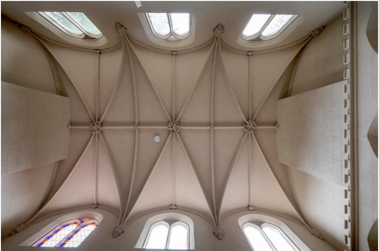
Cobham Dairy soon after completion in December 2019, and the restored vaulting in the central chamber.
