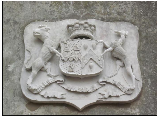
The Rolle Trefusis bearings before and after conservation, now with the animals' heads reinstated.
