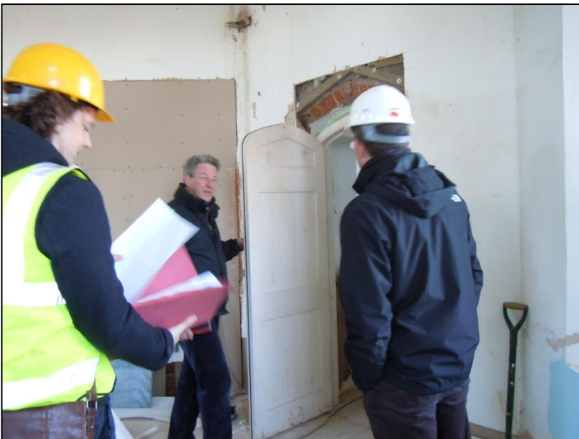
New doors of close grained pine carefully replicate the originals but must be constructed to comply with modern fire resistance regulations.
