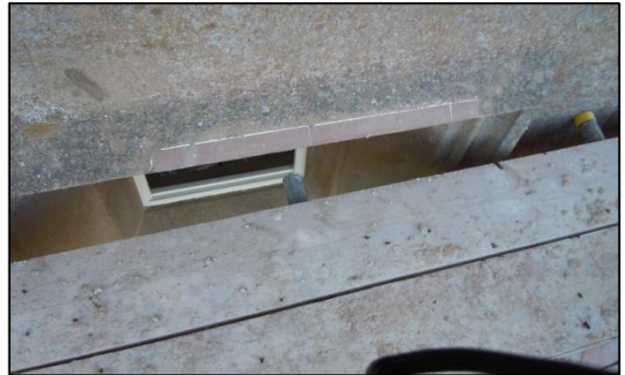
Examples of careful repair of the self-coloured render. The lichen is benign.
