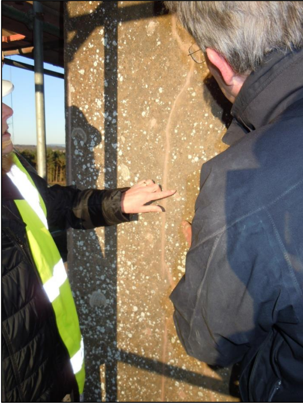
Examples of careful repair of the self-coloured render. The lichen is benign.
