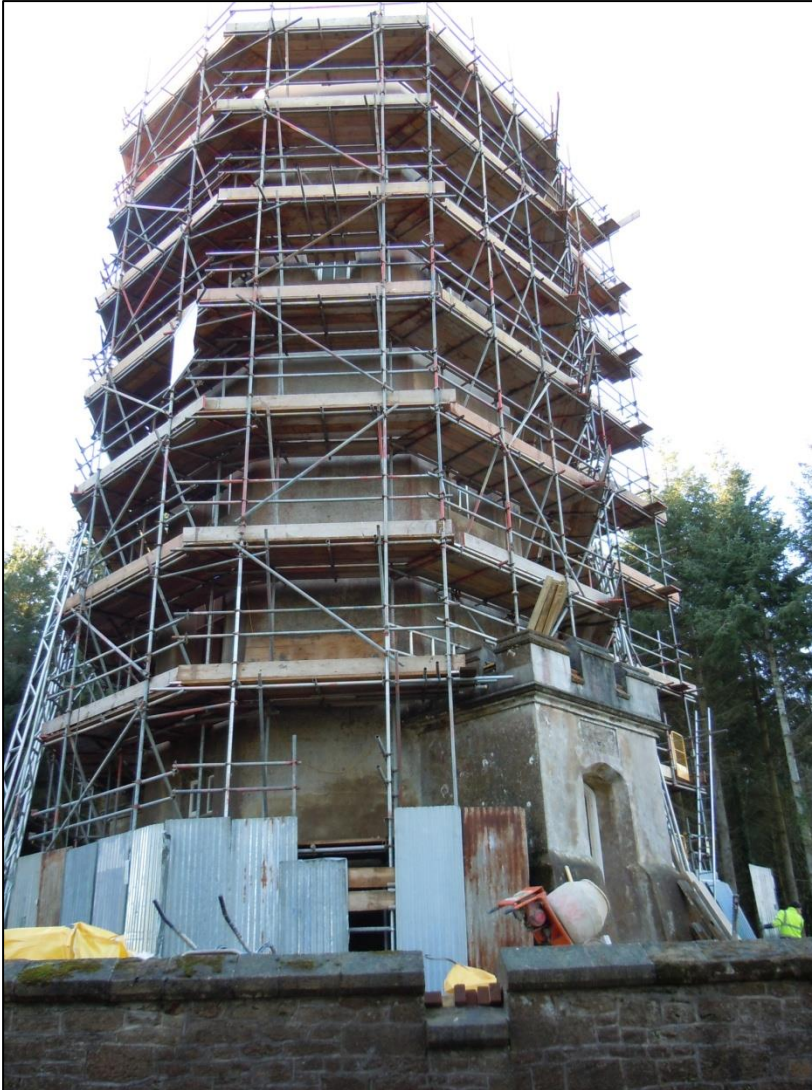
The tower was scaffolded from top to bottom during works.
