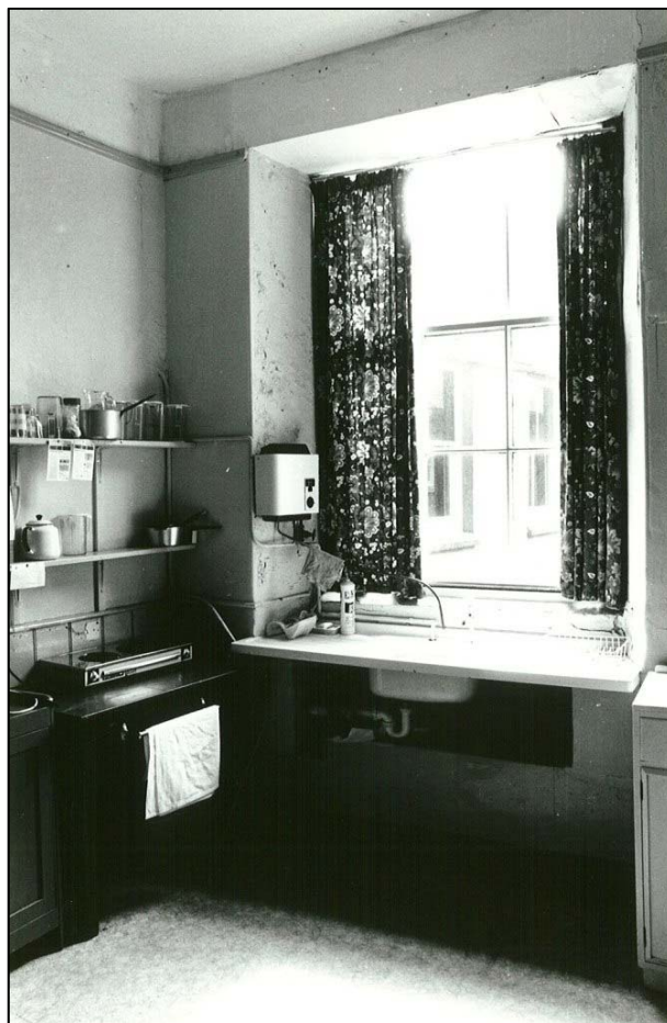
The Red Cross kitchenette. The position of the window has been changed.
