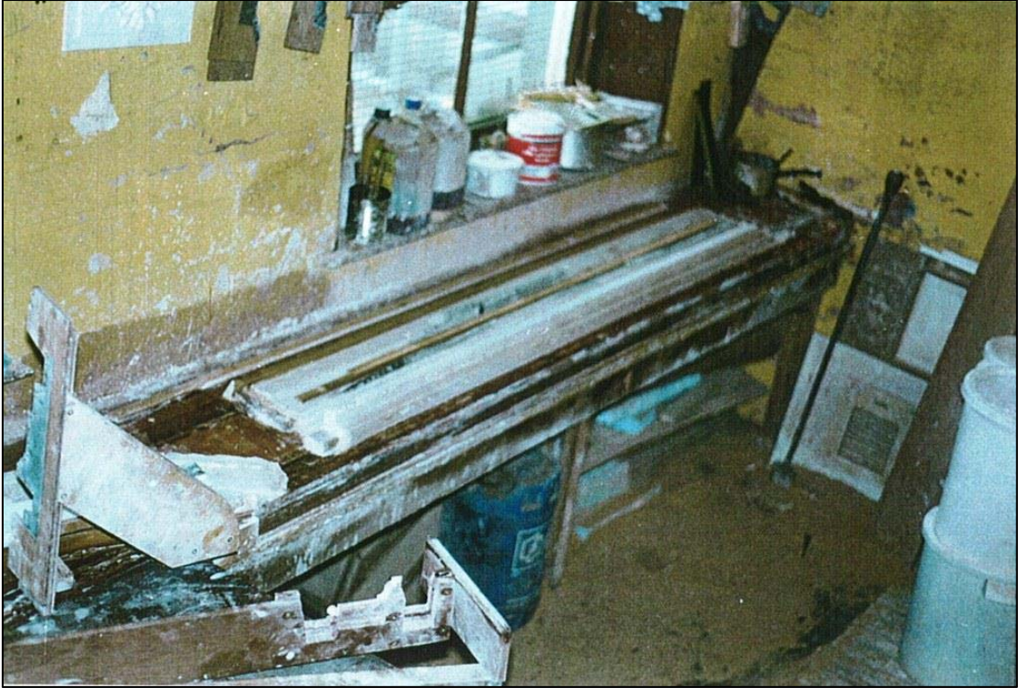
Plasterwork was remade on the workbench
