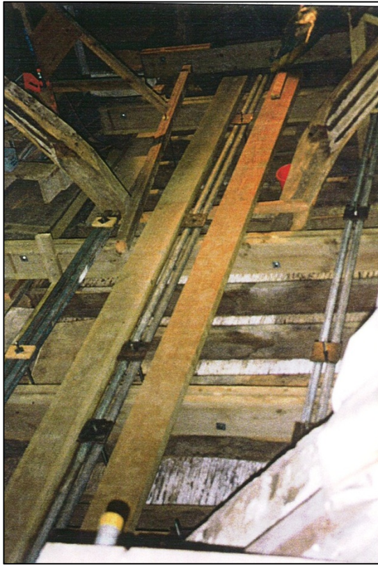
The centre gutter – note the cruck beams
