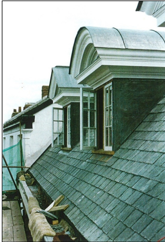
The dormers were remade and given lead roofs
