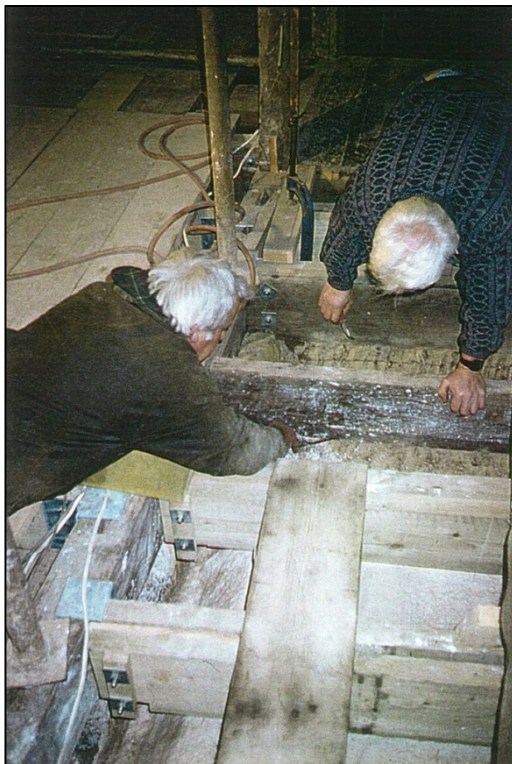
Working on the ceiling over the landing
