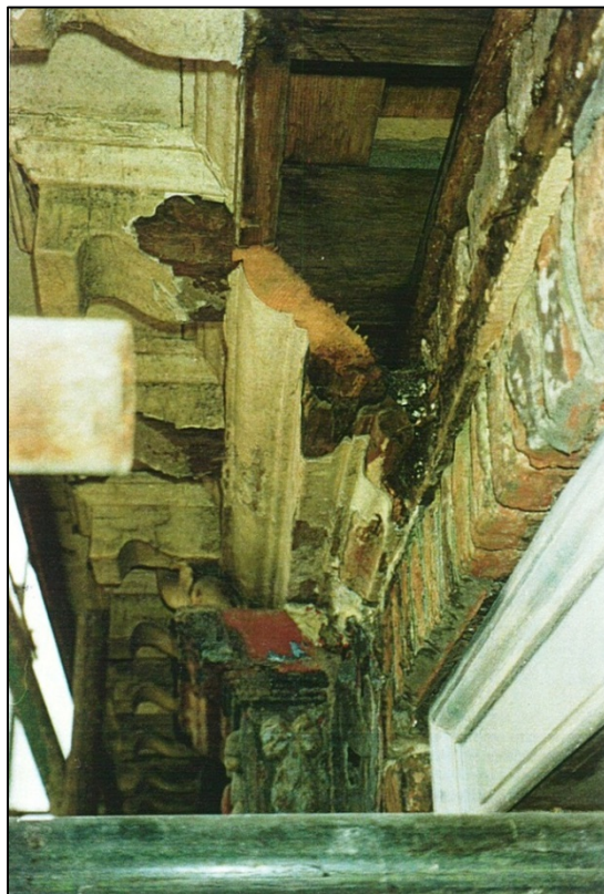
Rebuilding the cornice moulding
