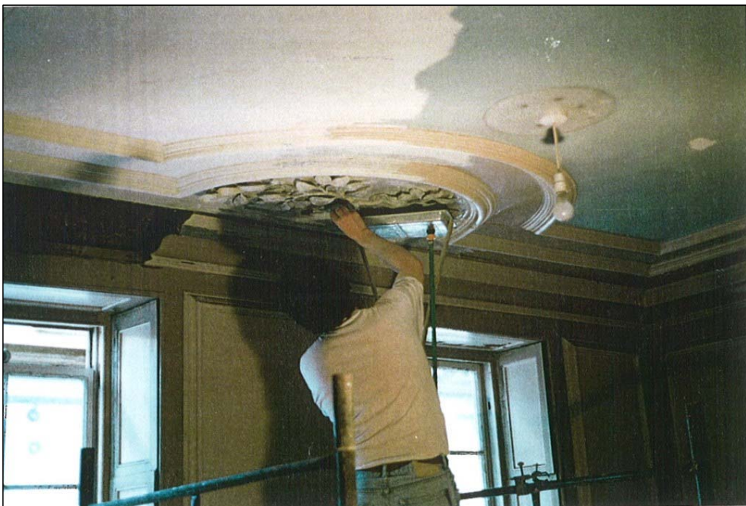
The ceiling in the north east bedroom being repaired
