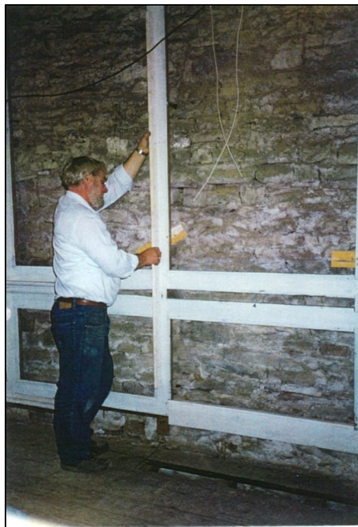
Relining the dining room wall
