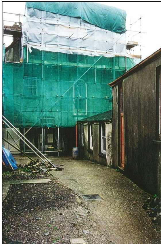
Work in progress at the back
