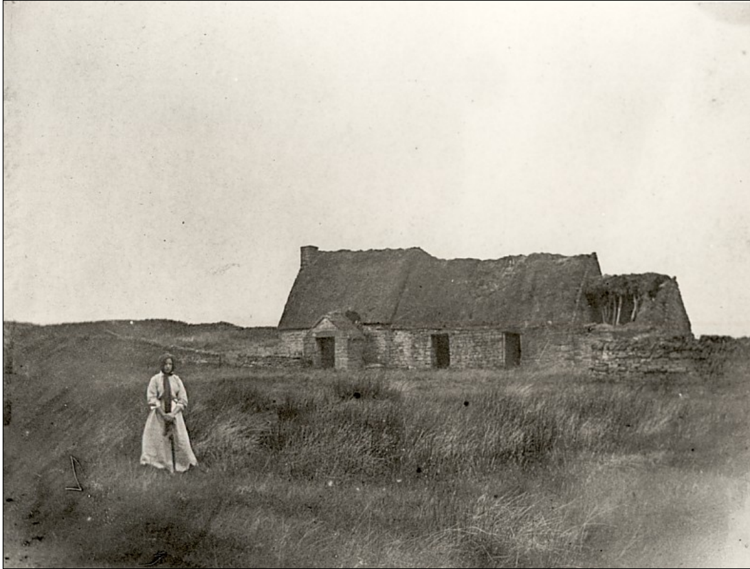
What almost happened to Causeway House: the gradual deterioration of Cragend, a heather-thatched steading not far away, recorded over some fifty or sixty years
