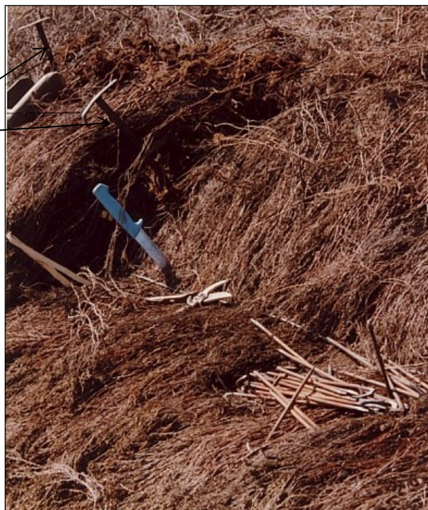
The ridge was dressed with a layer of turf green side up.
