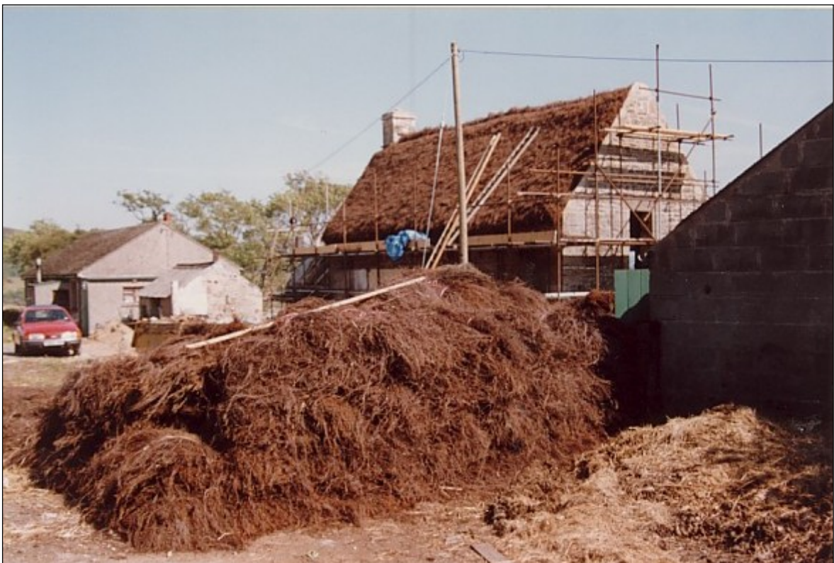
Thatching in progress during the summer 1989, before the bungalow was removed.
