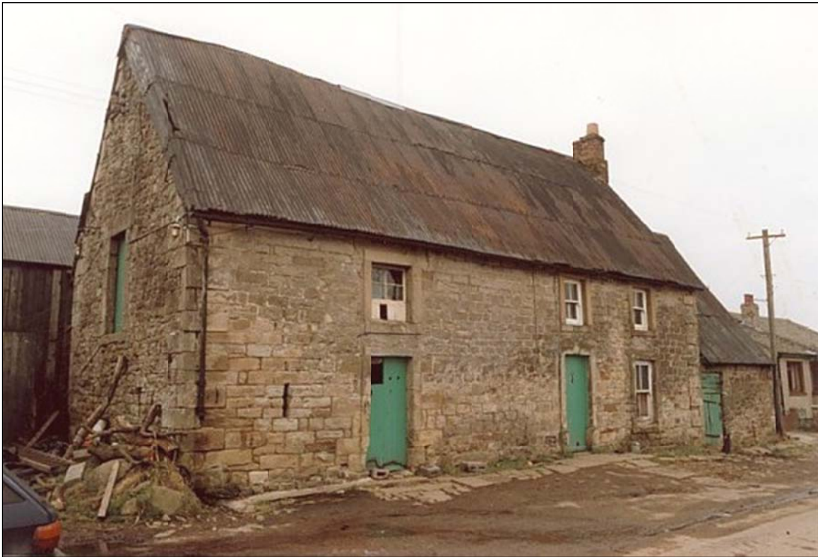
Causeway House in 1988, with its thatched roof covered with corrugated iron.
