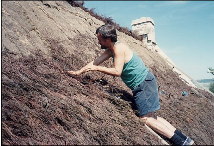
The turf under the thatch is laid green side down.
