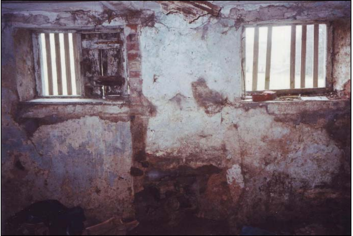
Note the surviving shutter. The glazing bars were modern, but one casement had survived.
