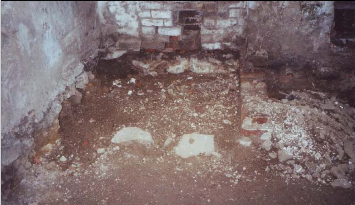
The earlier footings found beneath the kitchen floor.
