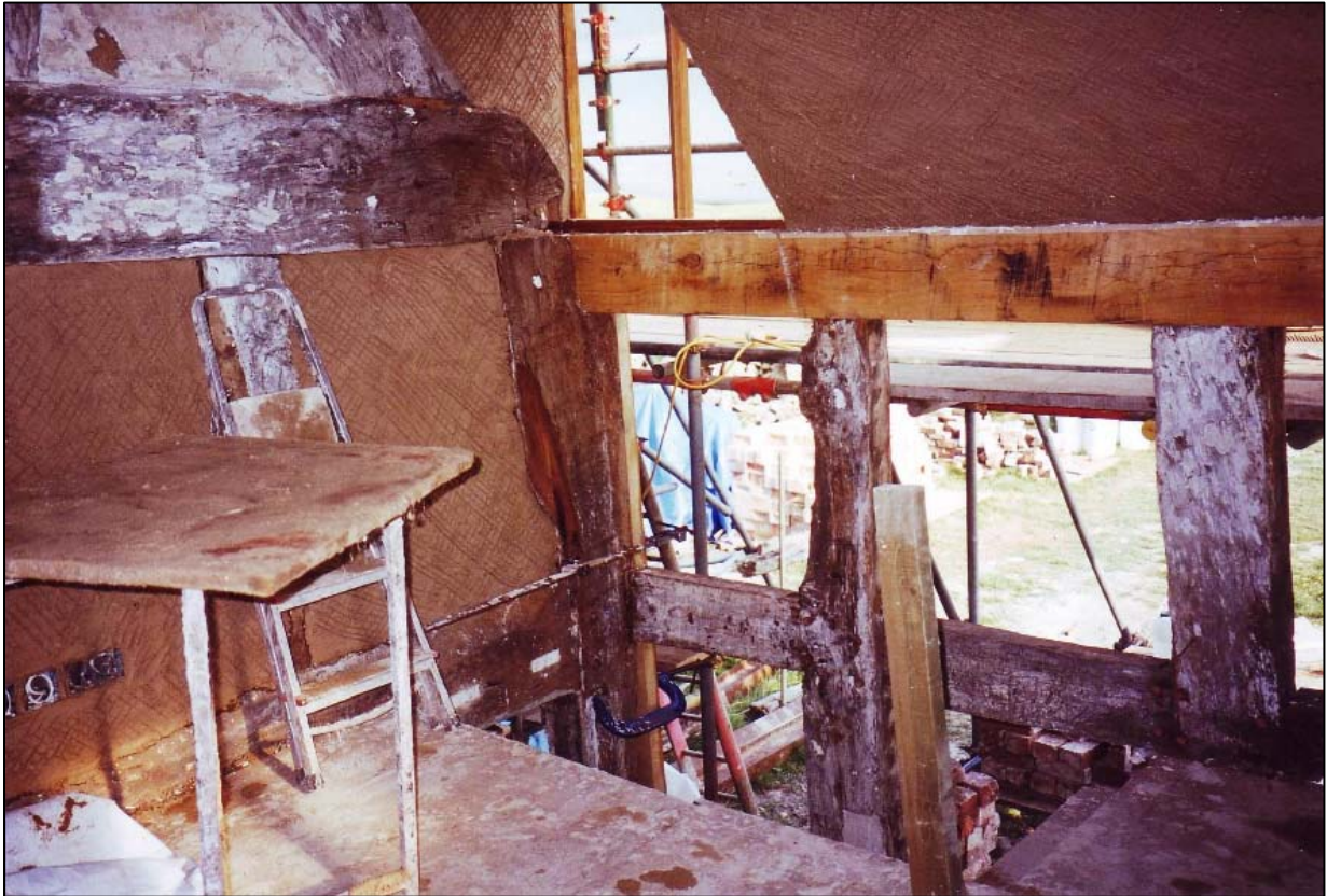
Scratch coat of lime mortar.
