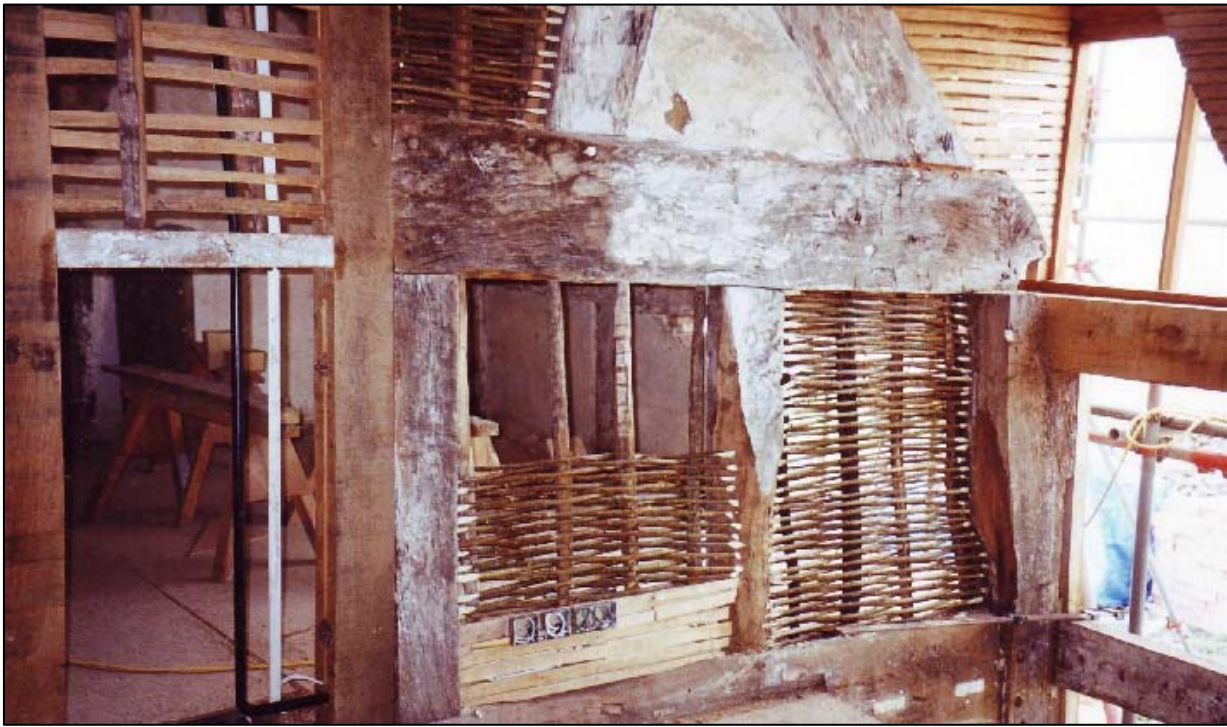
Just one panel could be salvaged in the first floor partition. Interweaved slender coppiced branches were used to renew the others, just as they would have been in the past – houseboote.
