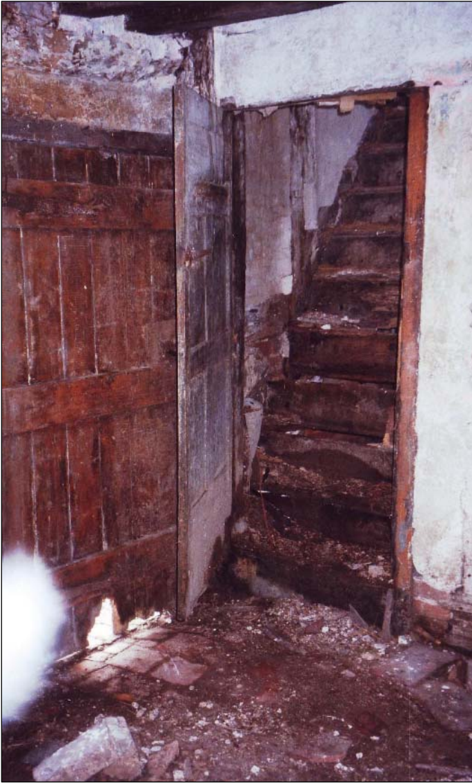
The elm stairs were too rotten to be saved, but like-for-like elm was used for their replacement, despite being hard to source since Dutch Elm Disease.
