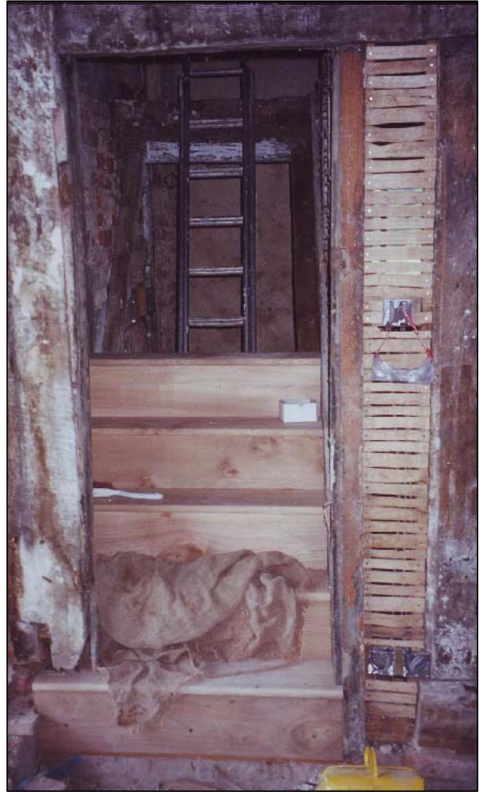
The elm stairs were too rotten to be saved, but like-for-like elm was used for their replacement, despite being hard to source since Dutch Elm Disease.
