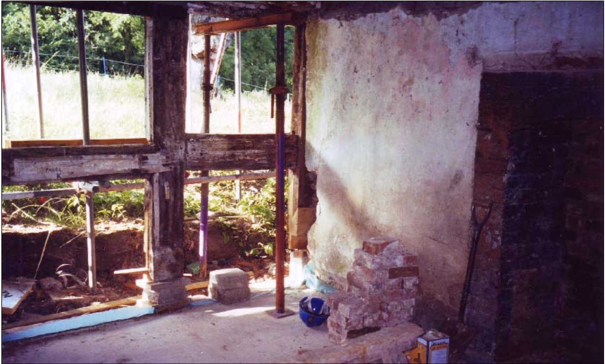
As much original fabric as possible was kept.
