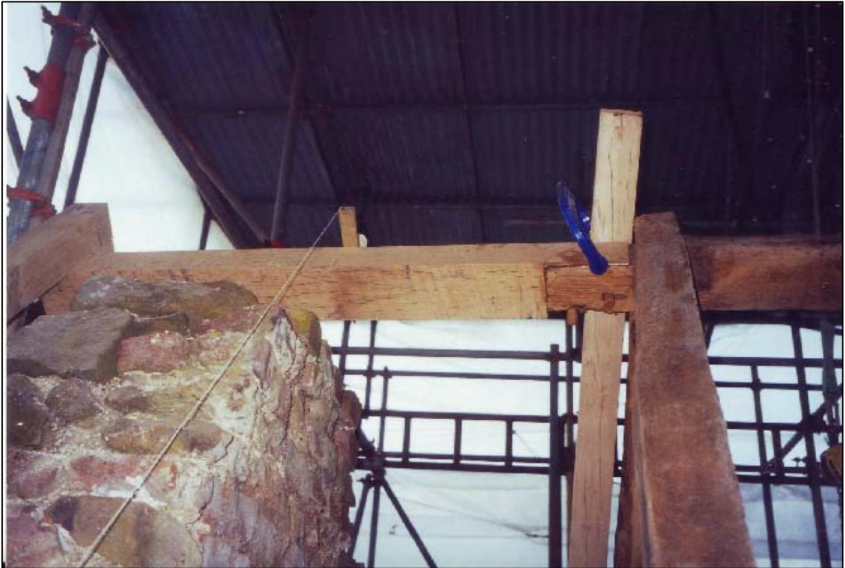
Replacement of the decayed end of the ridge pole, where it rests on one of the end gables. Most of the rafters had to have their chamfered ends replaced, and some had to be entirely renewed.
