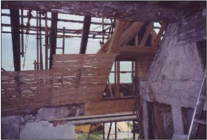
The dormer had to be renewed.
