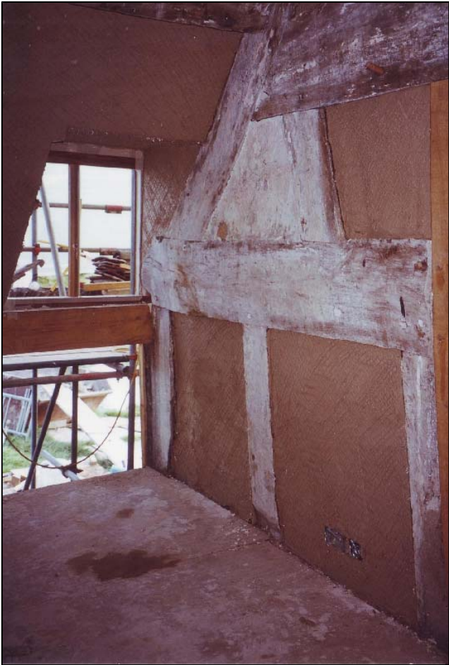
Just one panel could be salvaged in the first floor partition. Interweaved slender coppiced branches were used to renew the others, just as they would have been in the past – houseboote.
