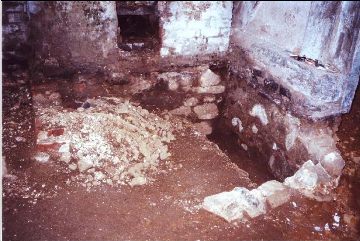
The earlier footings found beneath the kitchen floor.
