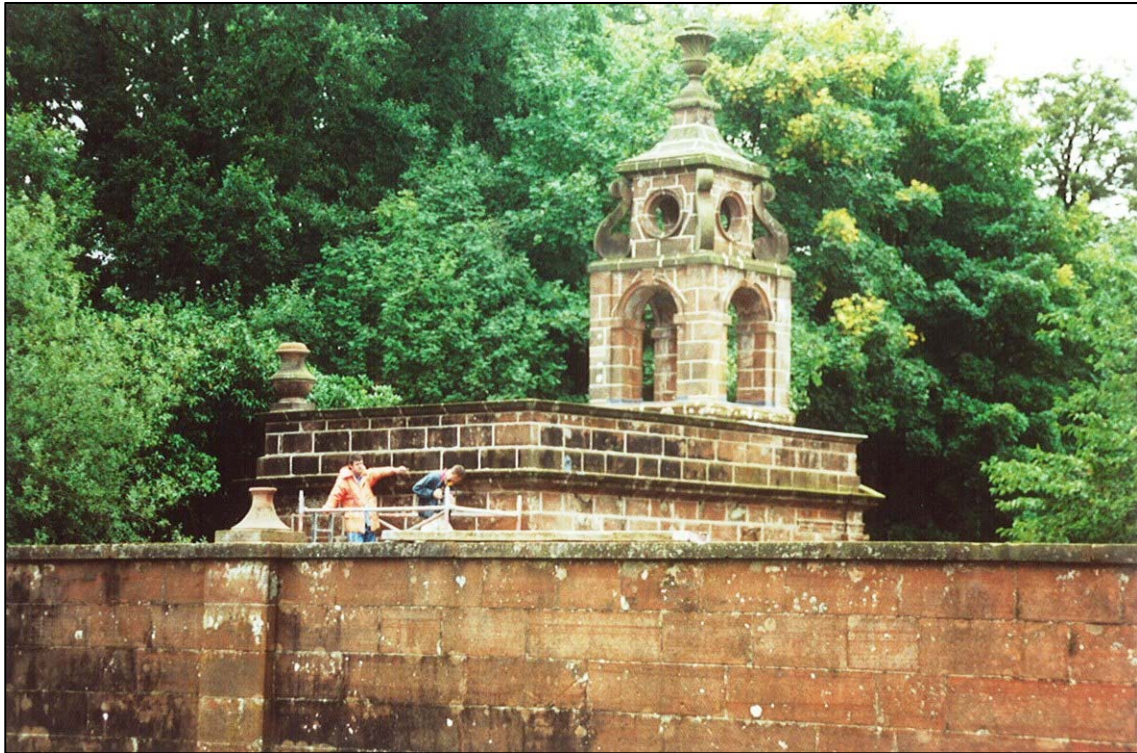
The South West Pavilion nearing the end of its restoration.
