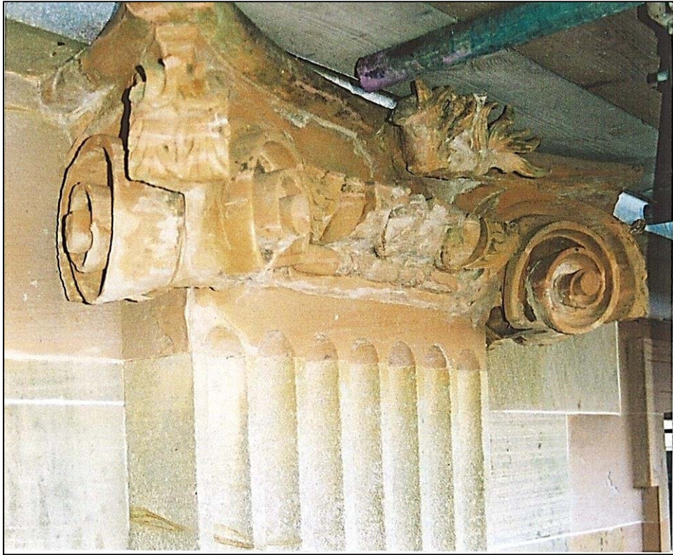
The fine capitals on the pilasters are more worn than they may appear. For now, we could not bear to compromise the original craftsmanship so they have been consolidated as found.
