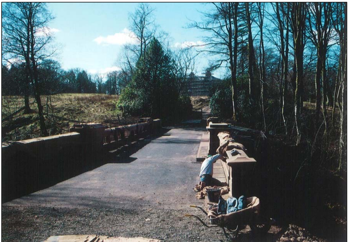
'Many hours pointing, re-pinning and grouting'
