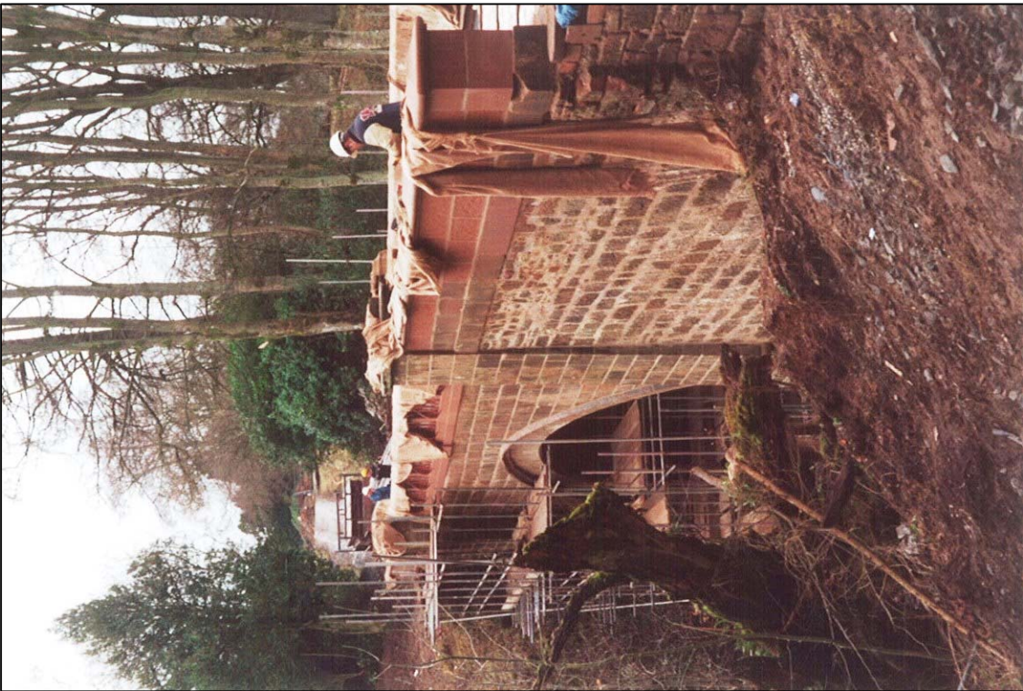
Repair work underway. The new cast iron balustrade and piers have been put back
