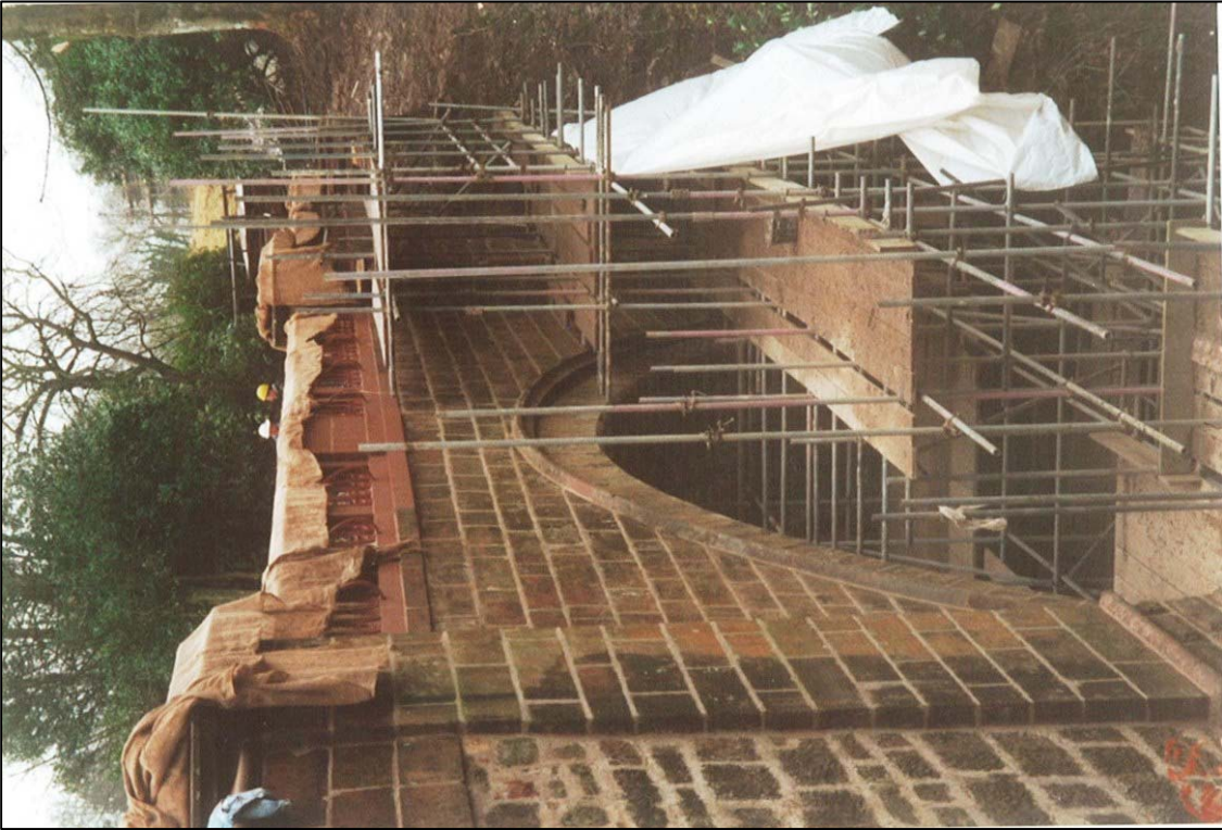
Repair work underway. The new cast iron balustrade and piers have been put back
