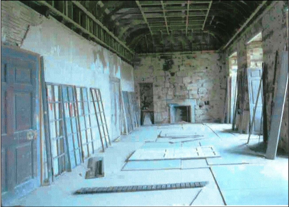
The library at the beginning of Landmark's involvement, completely stripped out with the ceiling structure reinstated by the SHBT. Crates of hand made mouldings stand waiting to replace the lost cornice (below).
