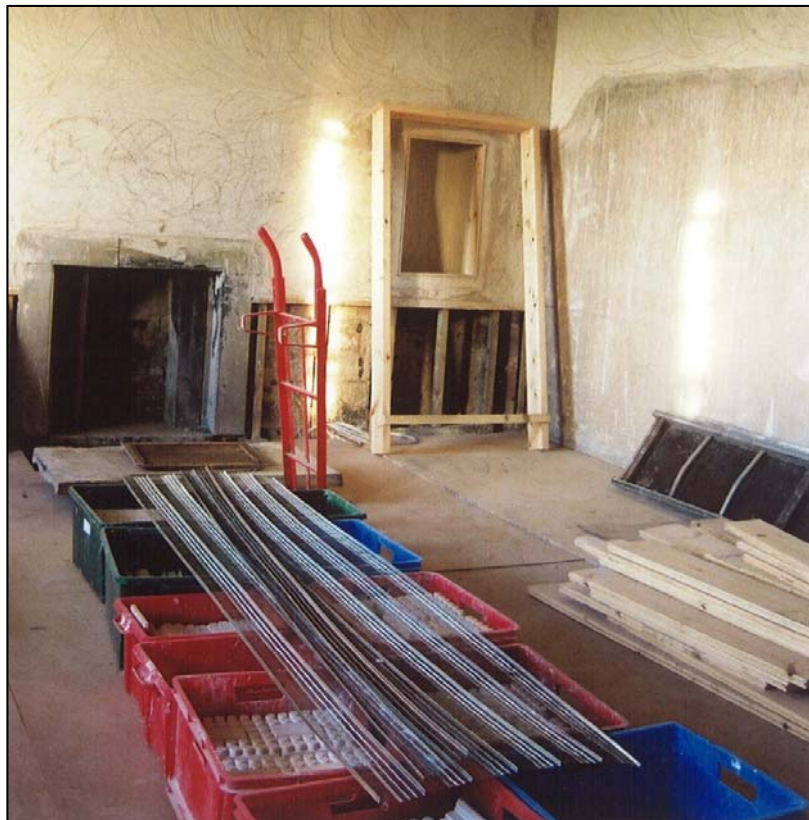
The library at the beginning of Landmark's involvement, completely stripped out with the ceiling structure reinstated by the SHBT. Crates of hand made mouldings stand waiting to replace the lost cornice (below).
