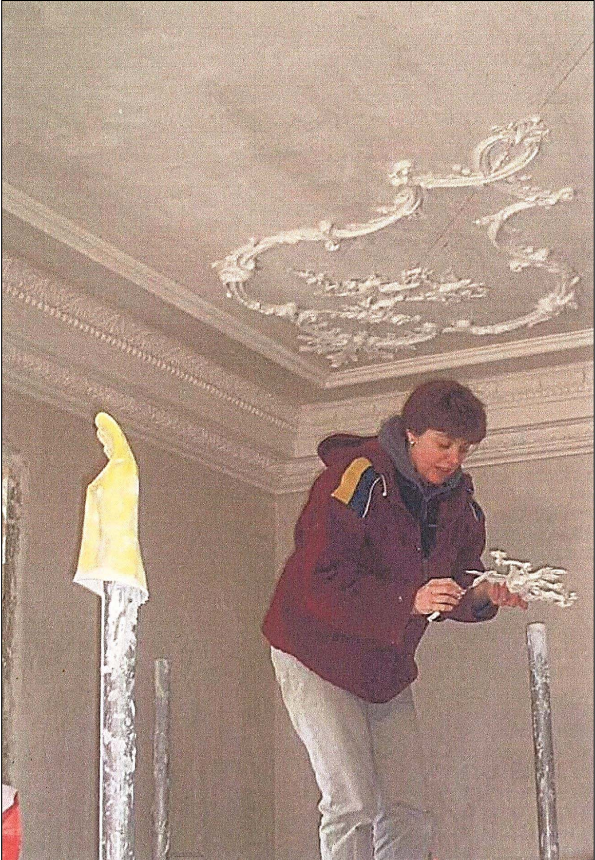
One of the Hirst Conservation team reinstating the damaged paper mache mouldings on the stairwell ceiling.
