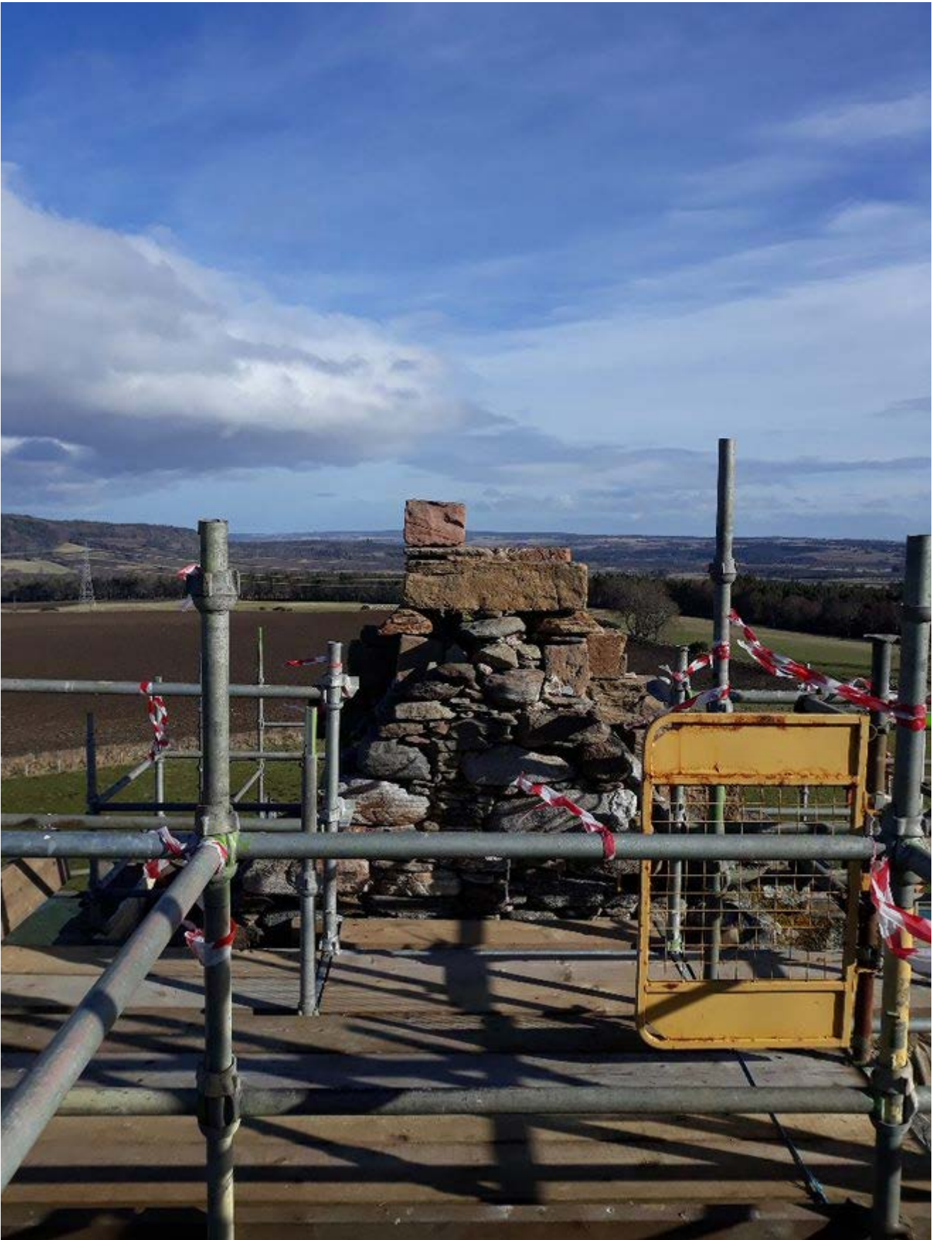
With the scaffolding in place, the views from the tower could finally be fully appreciated here at roof level.
