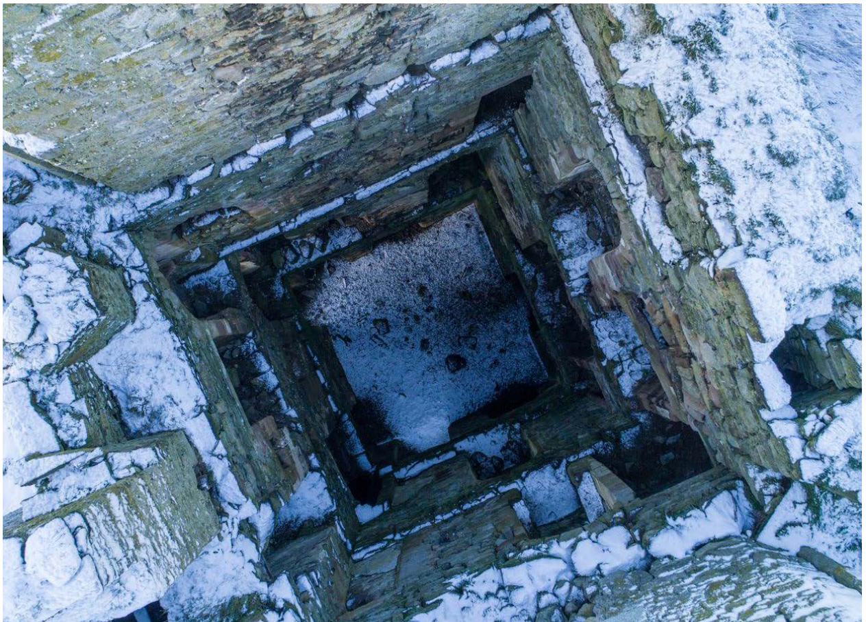
Drone shots of Fairburn Tower before restoration, in winter 2018. It stood as a completely gutted shell.
