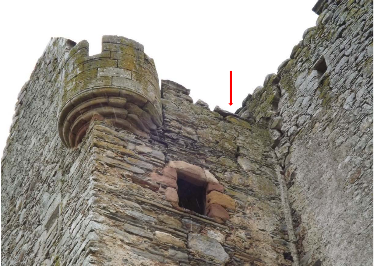
Upper parts of the early tower on the south side, showing the junction with the stair tower; location of former dormer window indicated.
