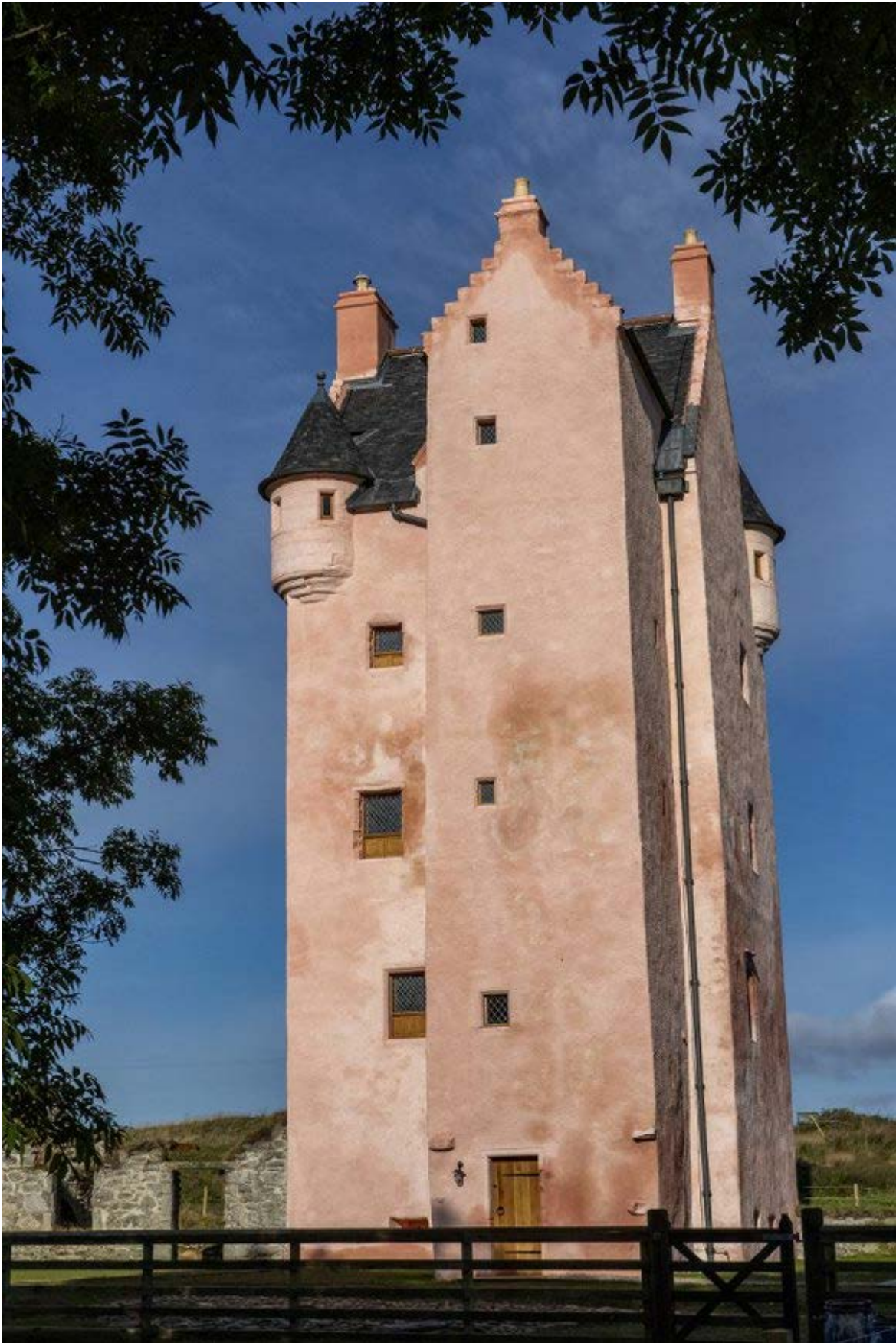
Fairburn Tower, newly completed in October 2022. (The damp patches on the exterior are caused by the differing porosity of stone beneath the render.)
