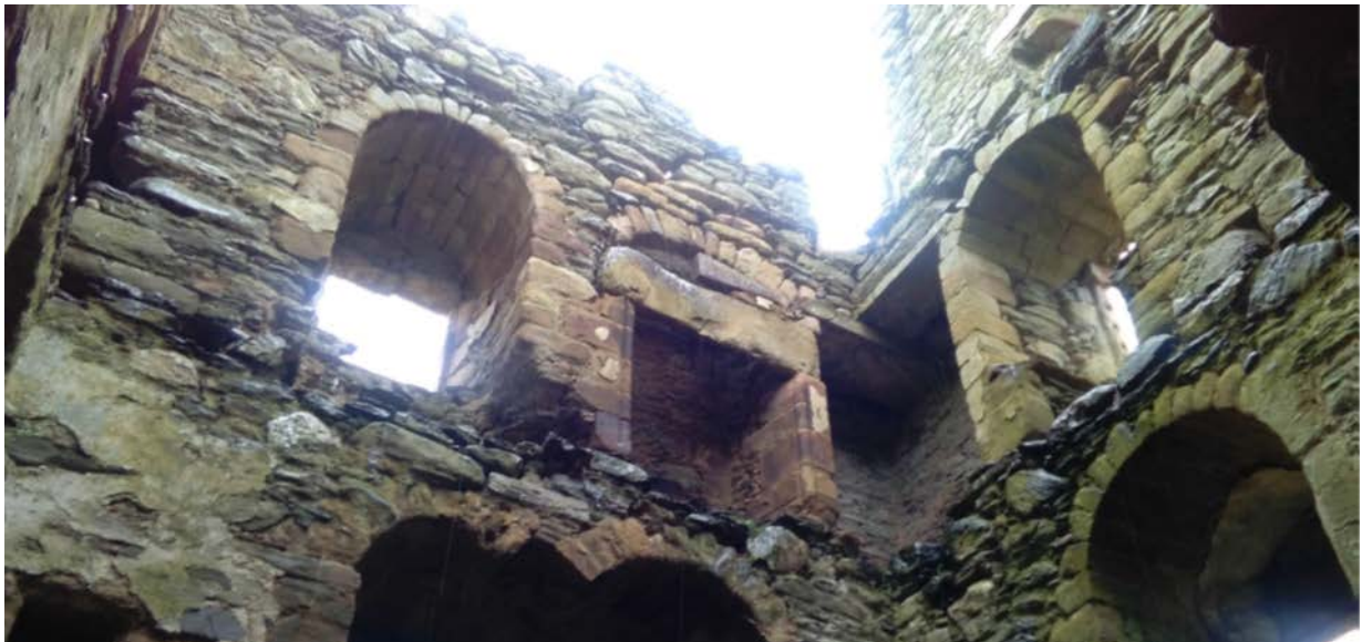
Third floor – interior arrangements to the north-east including fireplace and large mural recess at the angle.
