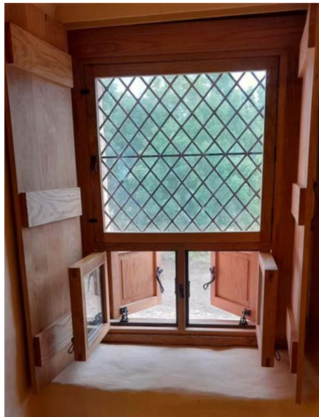
One of the flexible, practical shutter boarded windows.
