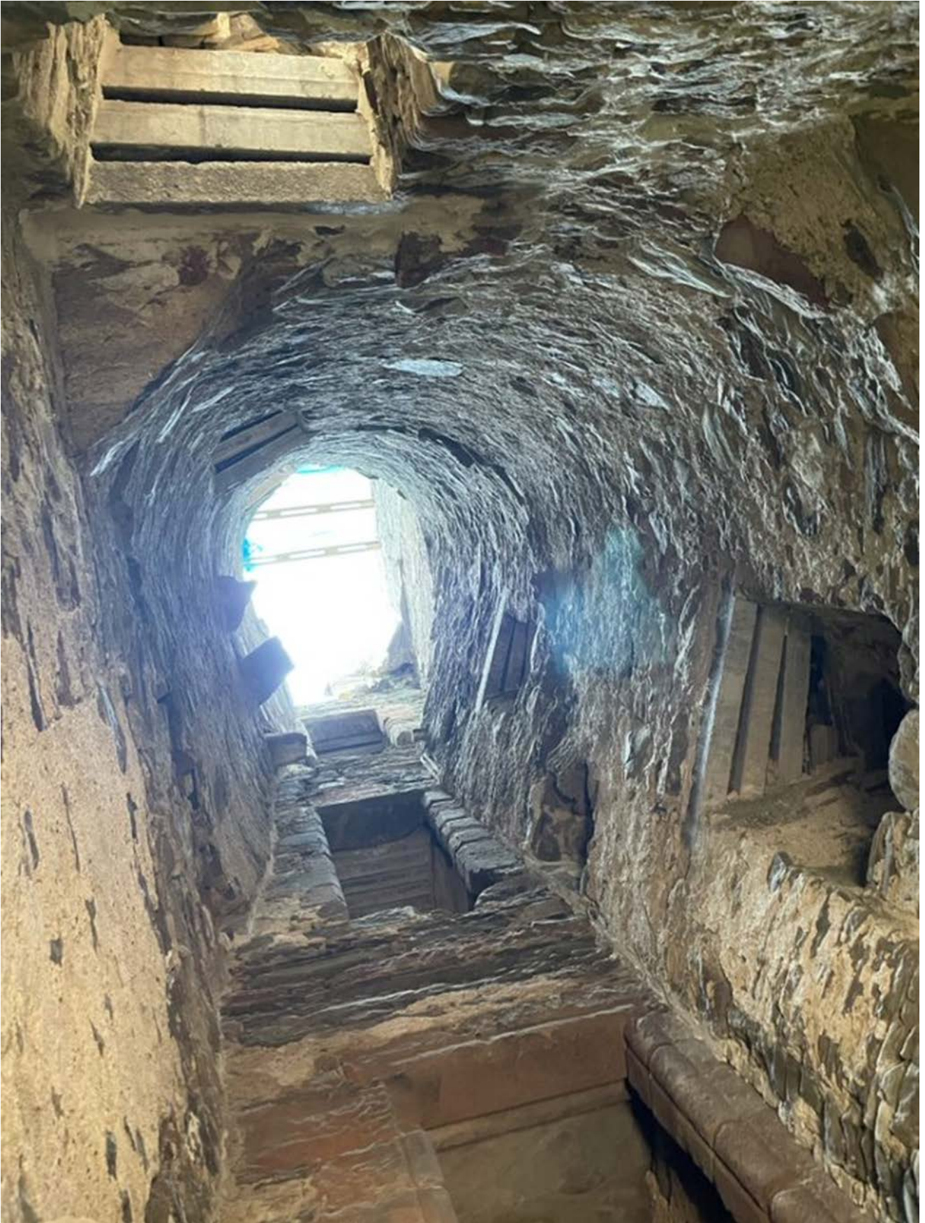
Interior of the stair tower.
