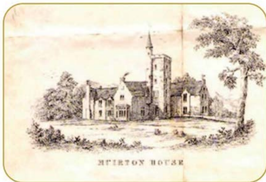
Muirton House in Wester Fairburn, demolished by John Stirling to make way for Fairburn House.
