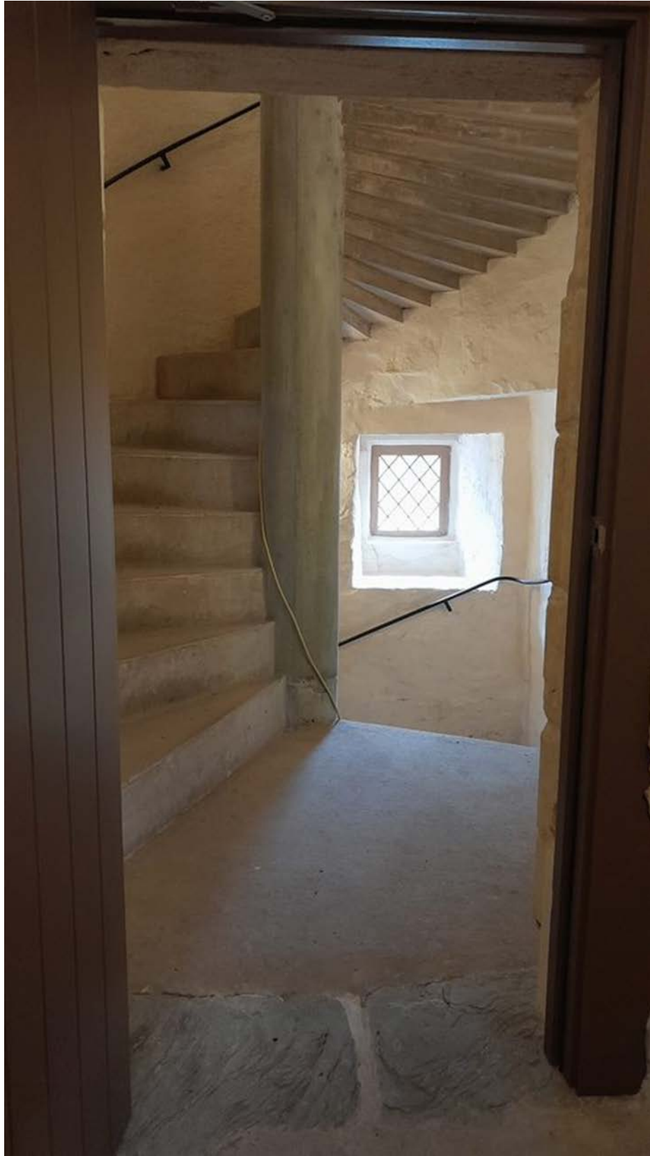
A section of the completed concrete stair.
