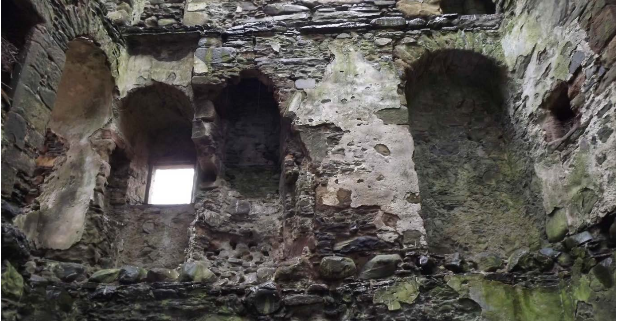
Occasional well-preserved areas of internal lime plaster survived, here at second floor level. These have been carefully incorporated into the new lime plaster where possible.
